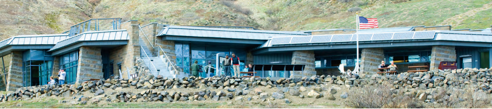
LEED Visitor Center, Denali National Park & Preserve, photo by Kent Miller
