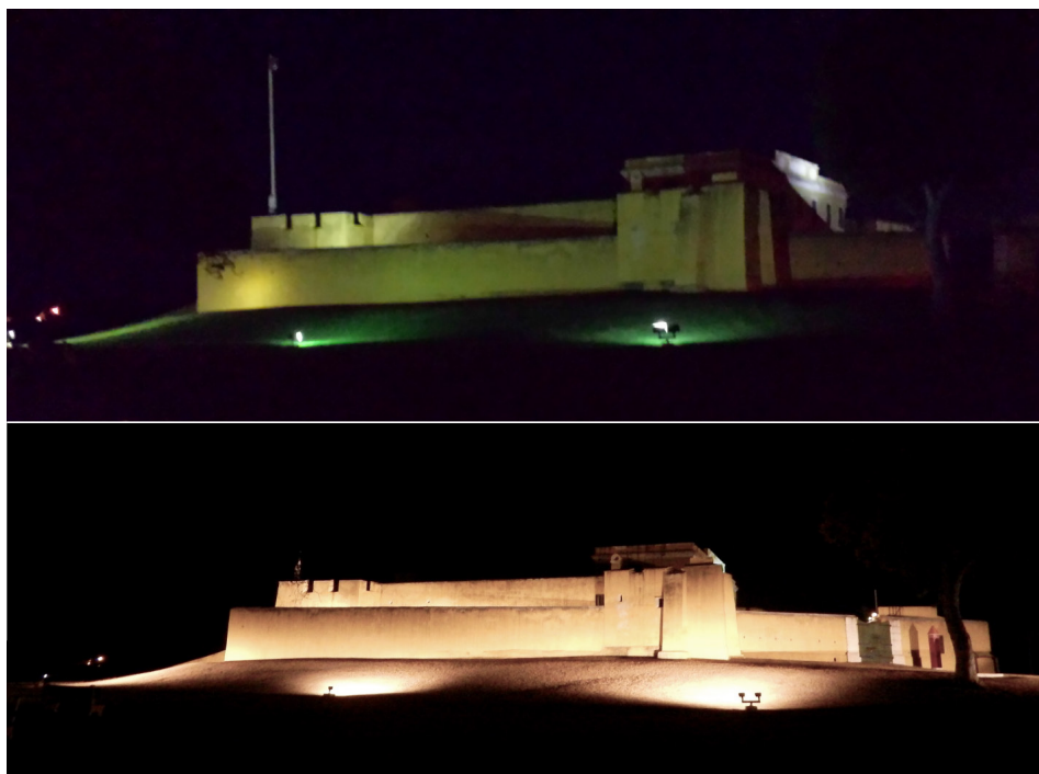
Fort Christianvaern, before and after lighting improvements.
