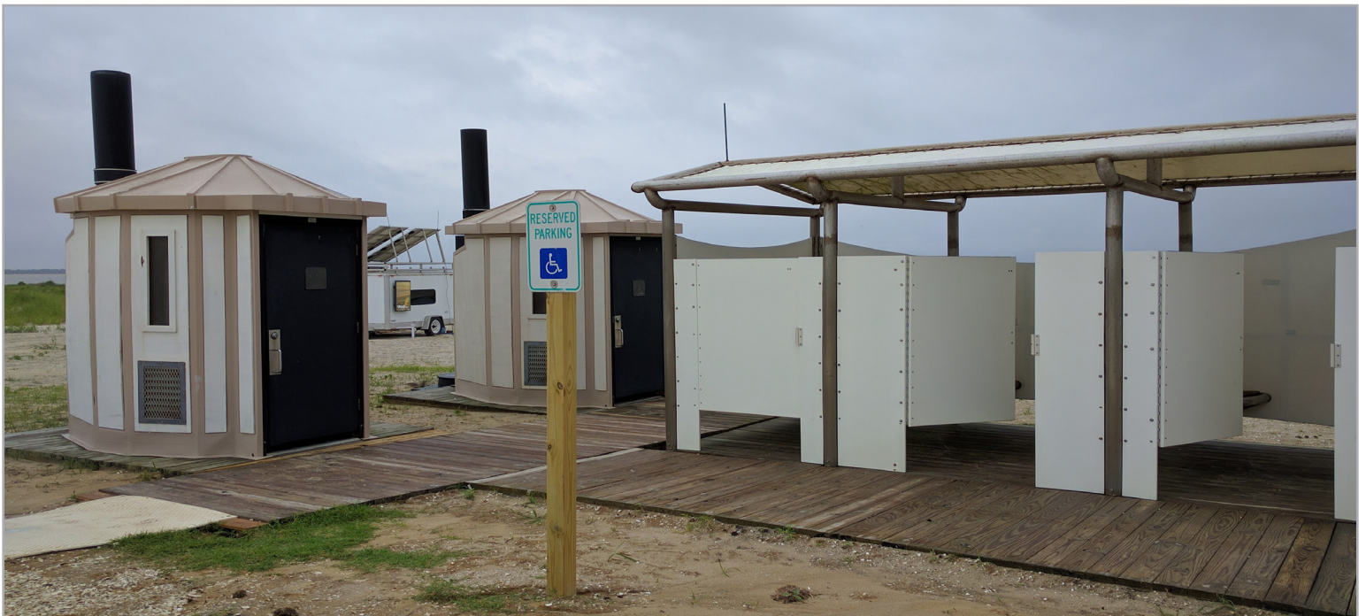
The utilization of moveable infrastructure along the beach helps manage risk and protect investments at Assateague Island National Seashore. NPS Image
