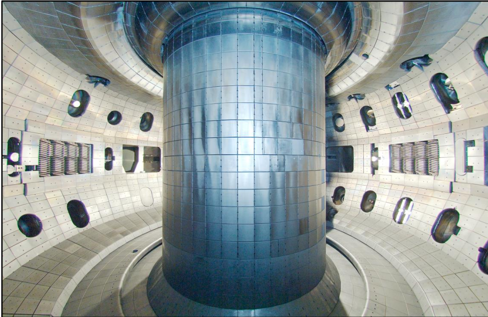
Interior of DIII-D vacuum vessel
