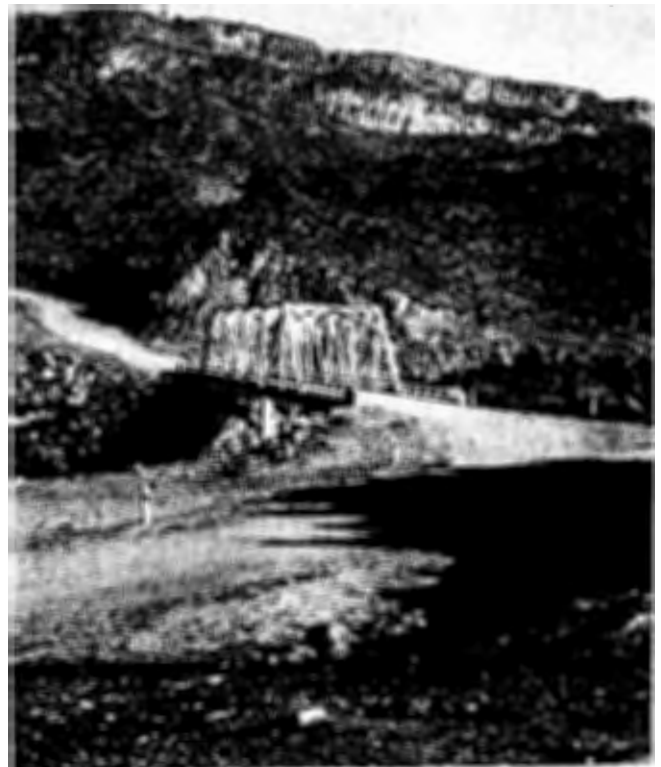
State Road 96 crossing at Taos Junction Bridge
