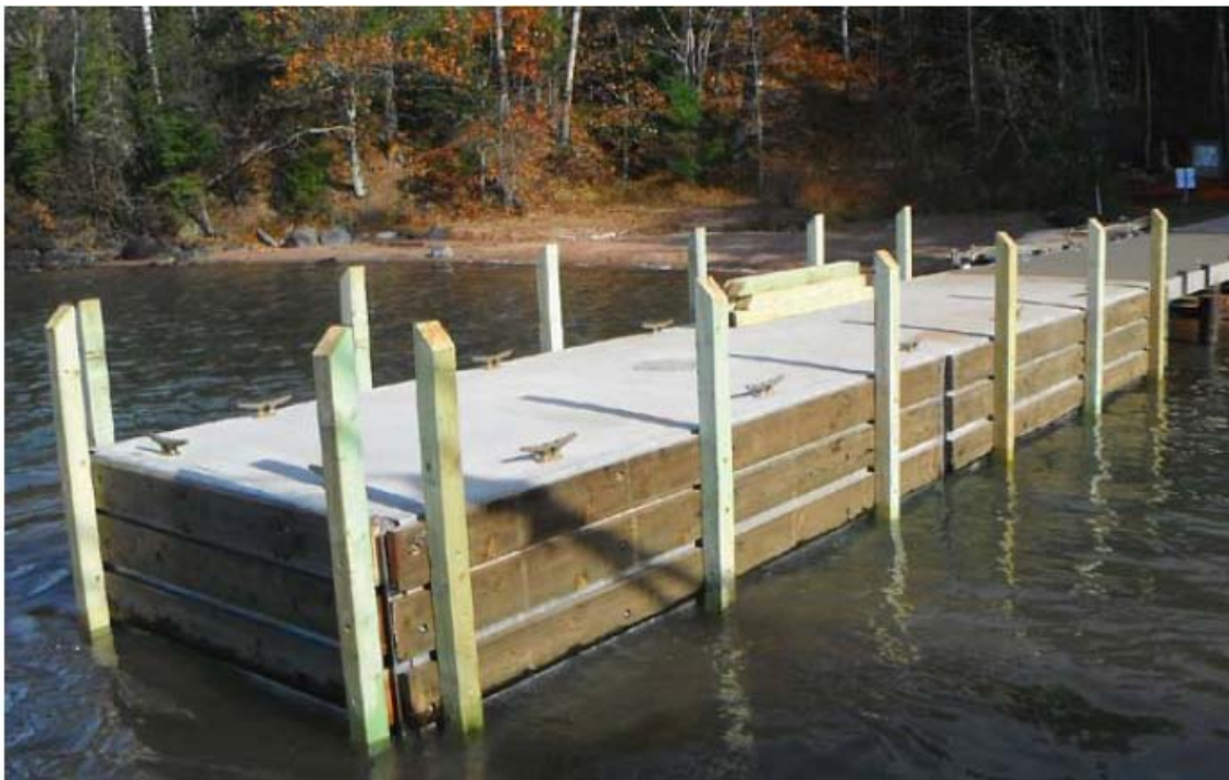
Basswood Island dock, Apostle Islands National Lakeshore. NPS photo.
