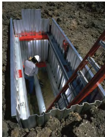
Photo courtesy of Speed Shore Corp.
