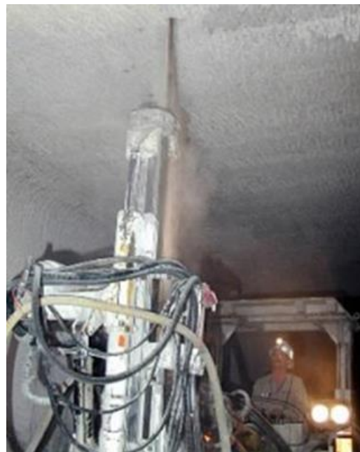
Figure 24: Roof Bolter Drilling to Install Roof Bolts
