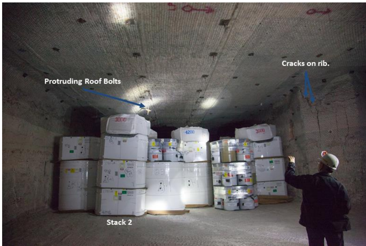
Figure 6: Active Waste Face at Panel 7 Room 7
