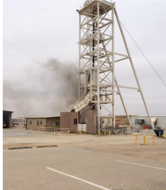
Figure 10: Smoke Visible Exiting through the Salt Shaft
