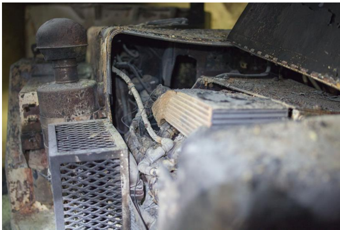
Figure 19: Engine Cooling Coils
