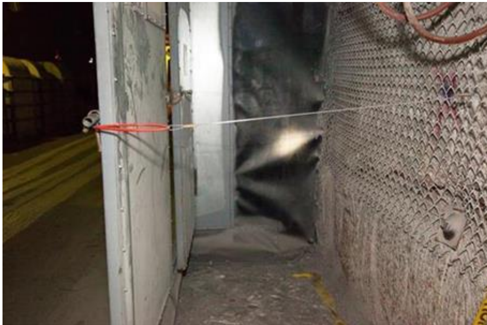
Figure 15: One of Chained Bulkhead Doors
