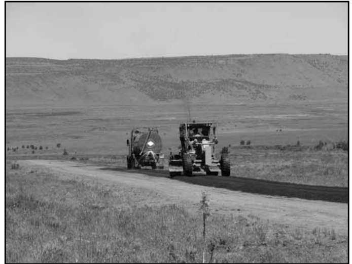
Photo R-2: Spreading New Surface Gravel on Roadway – Segment 11; June 28, 2010
