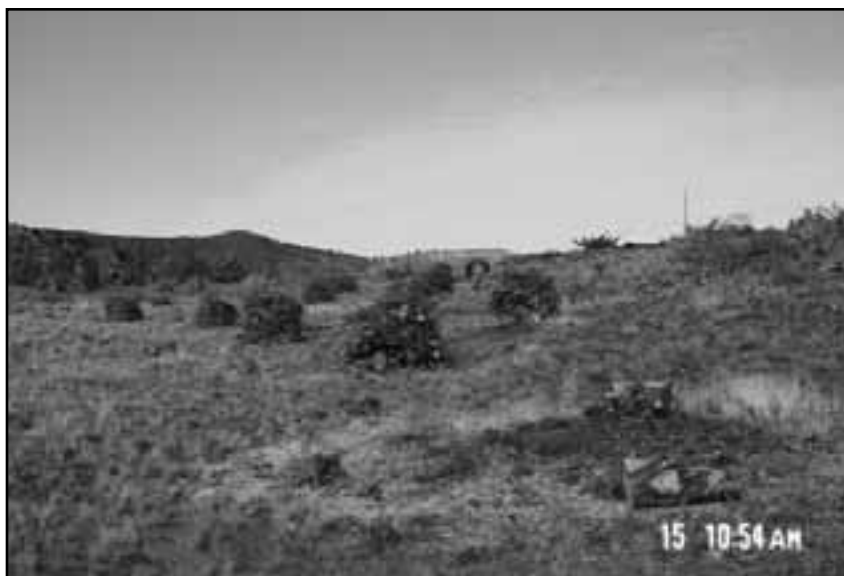
Photo WF-3: Contractor building handpiles above Frenchglen, OR
