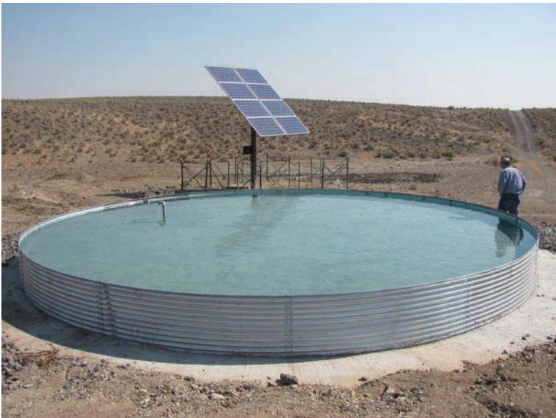
Pipeline Well New Trough
