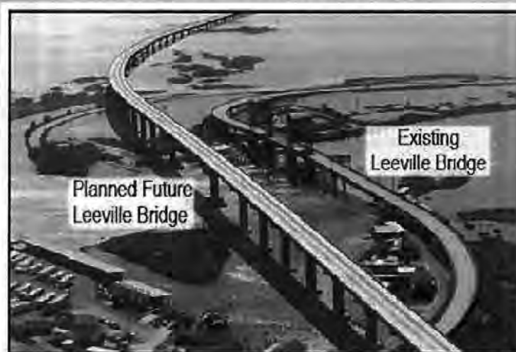
Figure 25.5. This “mock-up” shows the existing Highway LA-1 and Leeville Bridge in coastal Louisiana (on the right) with a planned new, elevated bridge that would retain functionality under future, higher sea level conditions (center left). (Current sea level and sinking bridge are shown here.) A 7-mile portion of the planned bridge has been completed and opened to traffic in December 2011. (Figure source: Greater Lafourche Port Commission, reprinted with permission).
