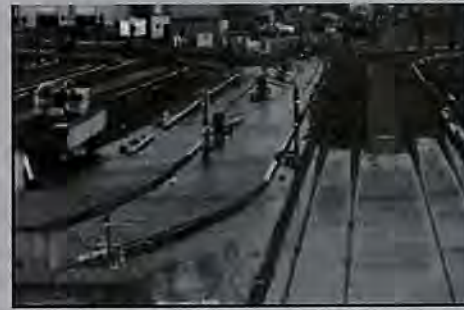
Figure 16.6. Flooded subway tracks in Coney Island after Hurricane Irene. (Photo credit: Metropolitan Transportation Authority of the State of New York 2011).
