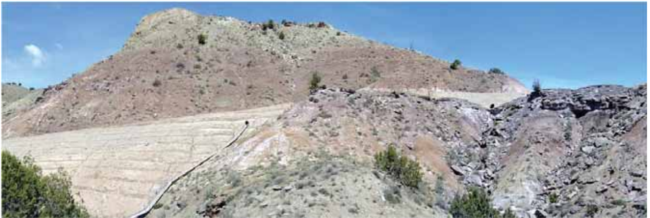
Siting this road on a side slope resulted in a large amount of fill that creates strong visual contrasts. (Credit: BLM.)
