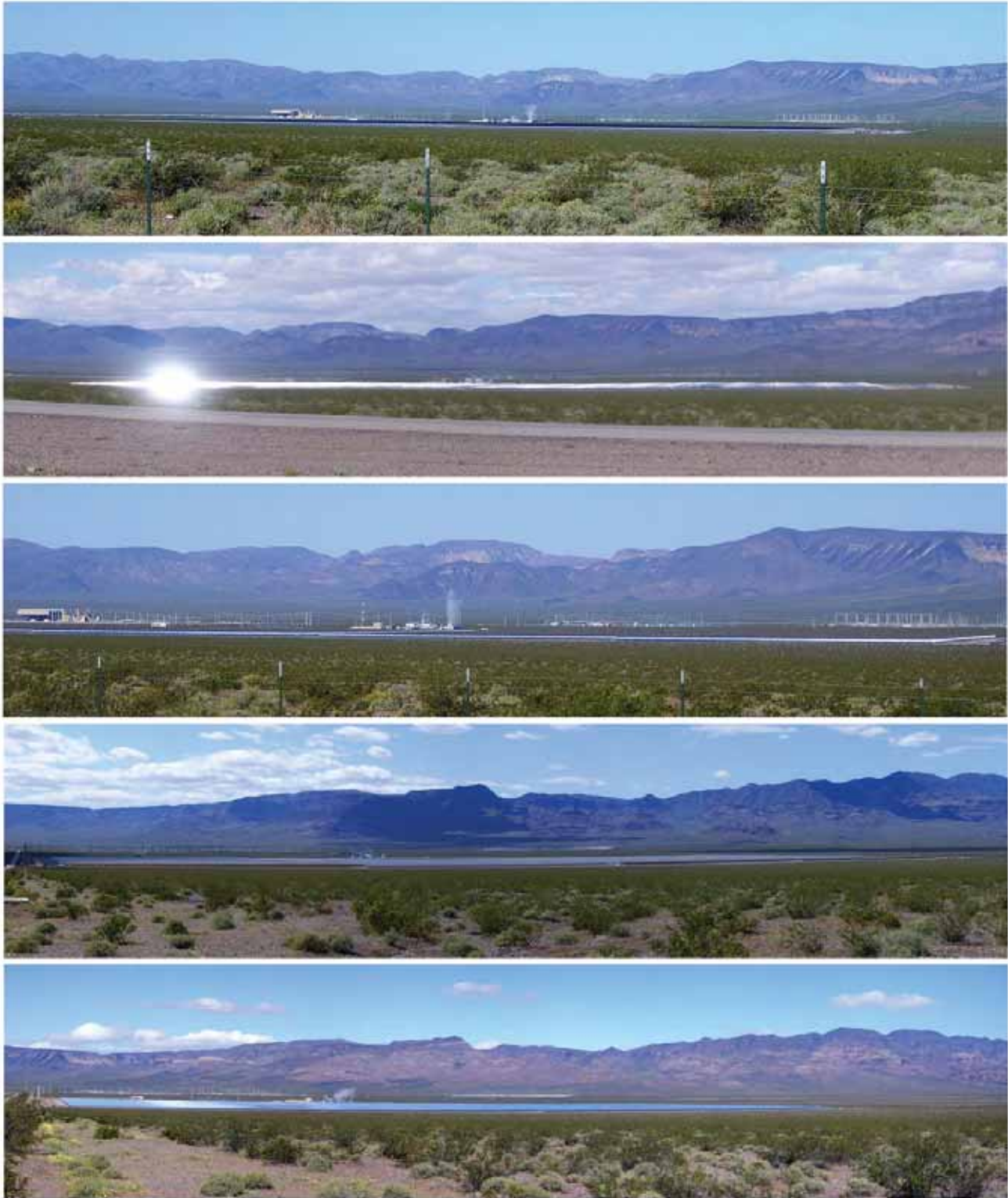
Effects of sun angle and lighting on parabolic trough facility color. The solar collector array can appear black, glittering silver-white, green, gray, or blue, as the mirrors reflect objects around them. (Nevada Solar One near Boulder City, Nevada. Credit: Robert Sullivan, Argonne National Laboratory.)
