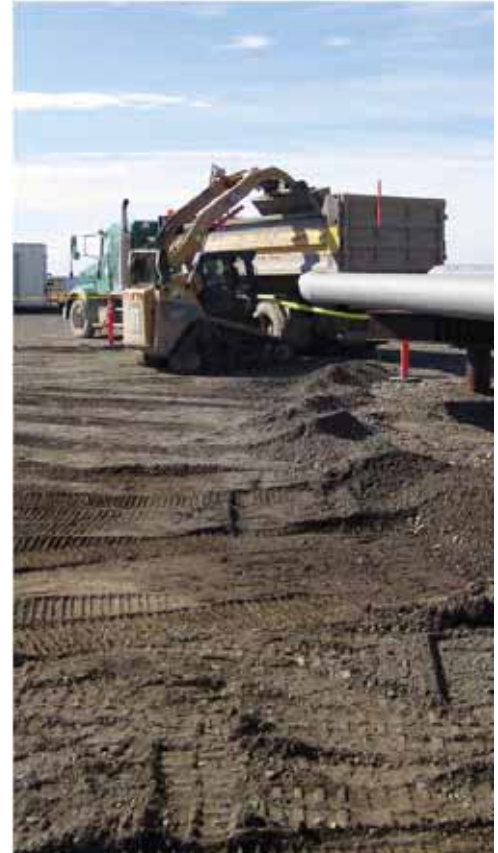
Gravel pad removal. (Credit: Alaska Department of Environmental Conservation.)
