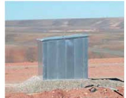
This untreated galvanized structure contrasts strongly with its surroundings and is also a potential source of strong glare. (Credit: BLM.)
