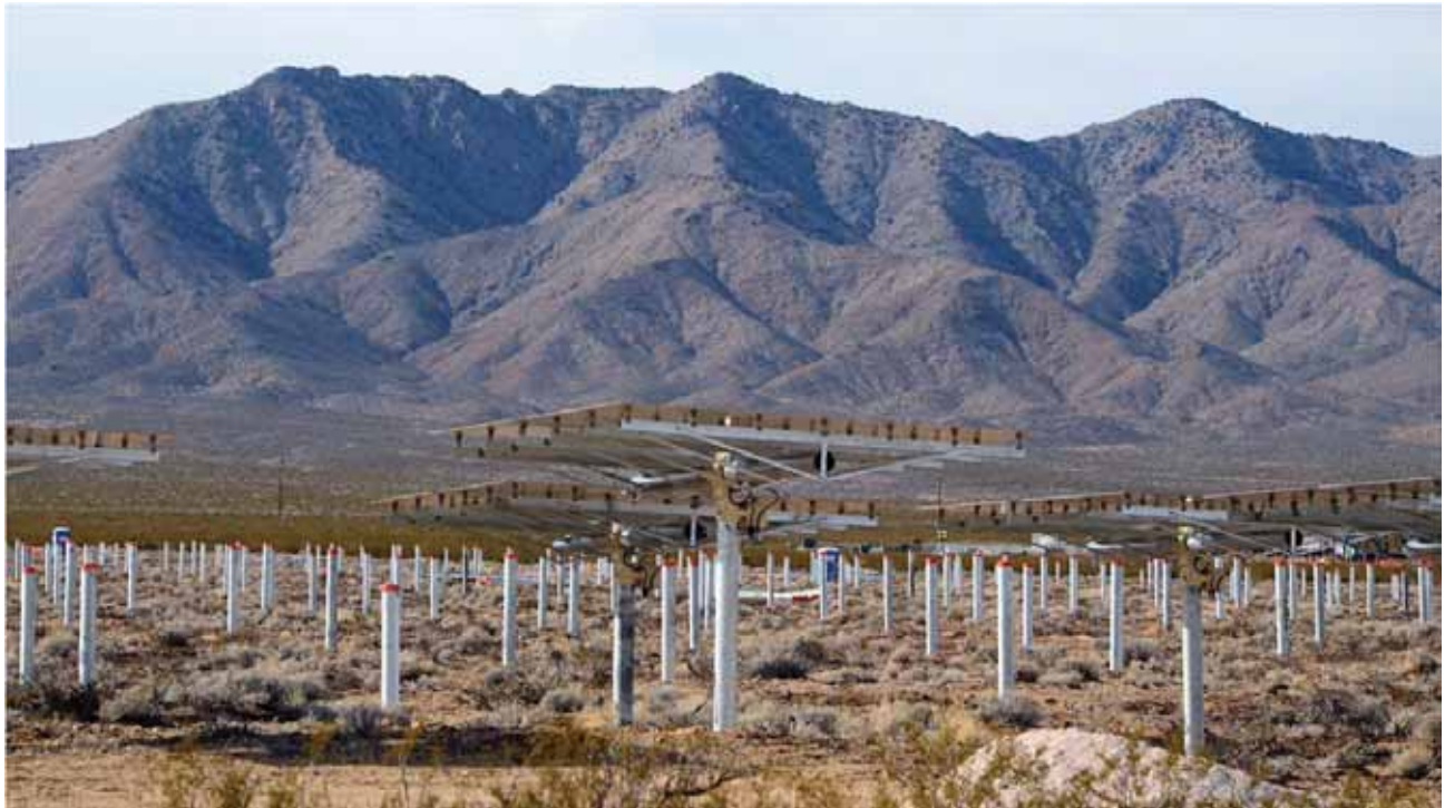
Trimmed vegetation beneath power tower heliostats (facility under construction). (Ivanpah SEGS facility, Ivanpah Valley, California. Credit: Robert Sullivan, Argonne National Laboratory.)
