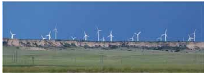
Viewed from the west, a dark cloud backdrop behind wind turbines illuminated by late afternoon sun results in very high visual contrast. (Cedar Creek Wind Farm, near Grover, Colorado. Credit: Robert Sullivan, Argonne National Laboratory.)
