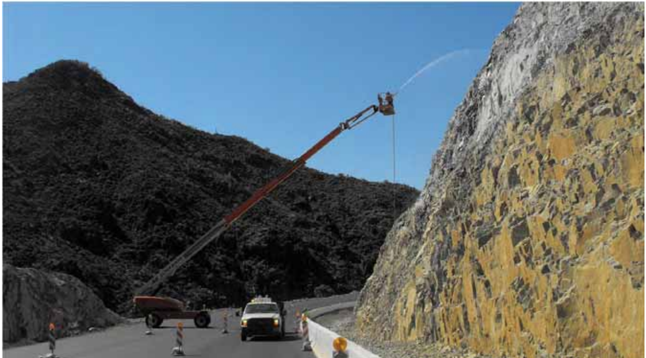
Application of oxidizing color treatment on excavated rock face. (Credit: Craig Johnson, Logan Simpson Design, Inc.)
