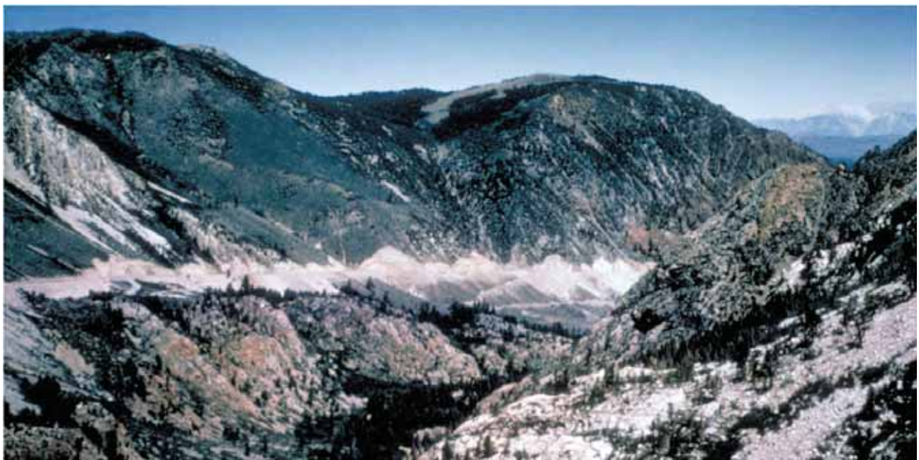
Building this road on a steep side slope resulted in excessive and highly visible cut and fill. (Credit: BLM)
