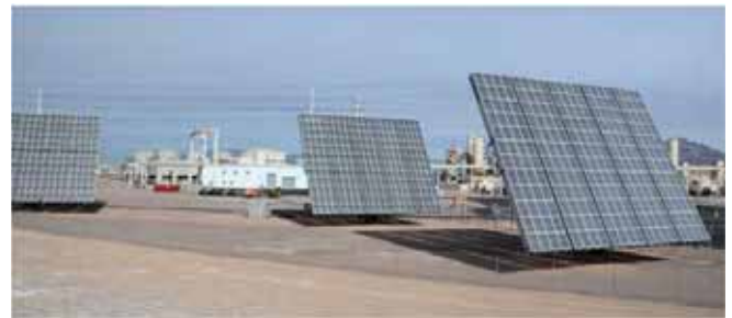
CPV units on dual-axis trackers. (Clark Generating Station, Las Vegas, Nevada. Credit: Robert Sullivan, Argonne National Laboratory.)
