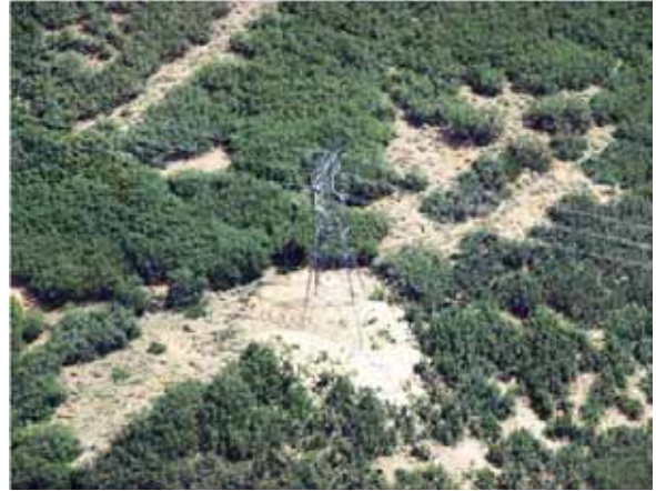
The clearing for the transmission tower was shaped to blend in well with the naturally occurring clearings in the surrounding area. (Credit: BLM.)
