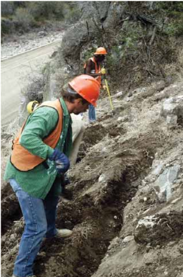
Preparing furrows along a slope to plant bare-root stock. (Credit: John McCarty, Colorado Department of Transportation.)
