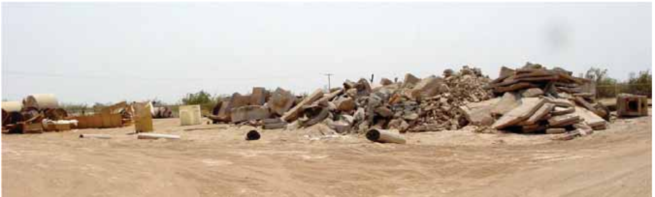
Debris pile at an operating geothermal plant creates an eyesore. (Credit: BLM.)
