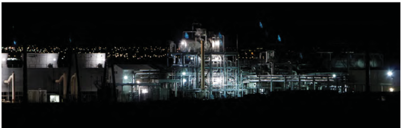
Nighttime shot of the power block and part of the cooling tower at a solar parabolic trough facility. Bright lights combined with many complex, highly reflective surfaces makes this facility lighting easily visible at distances greater than 10 mi (Nevada Solar One, near Boulder City, Nevada. Credit: Marc Sanchez, BLM.)
