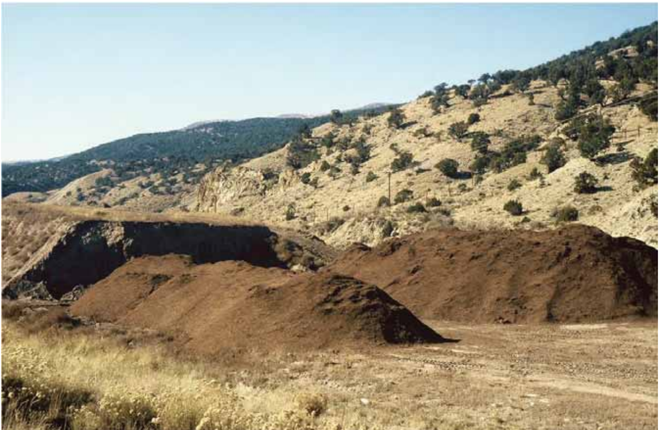
Stockpiled topsoil. In this case, composted sewage sludge (two darker piles in foreground) was mixed with soil from the topsoil stockpile behind and to the left of the mixed soil/compost piles. (Credit: John McCarty, Colorado Department of Transportation.)
