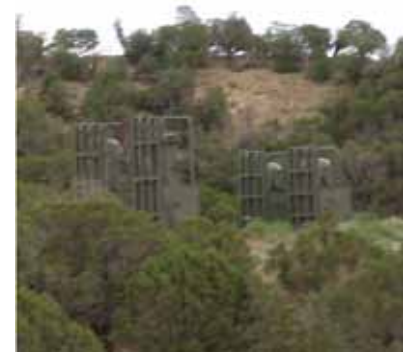
These structures have been painted with a BLM standard environmental color, and are difficult to distinguish from the surrounding vegetation. (Credit: John McCarty, BLM.)
