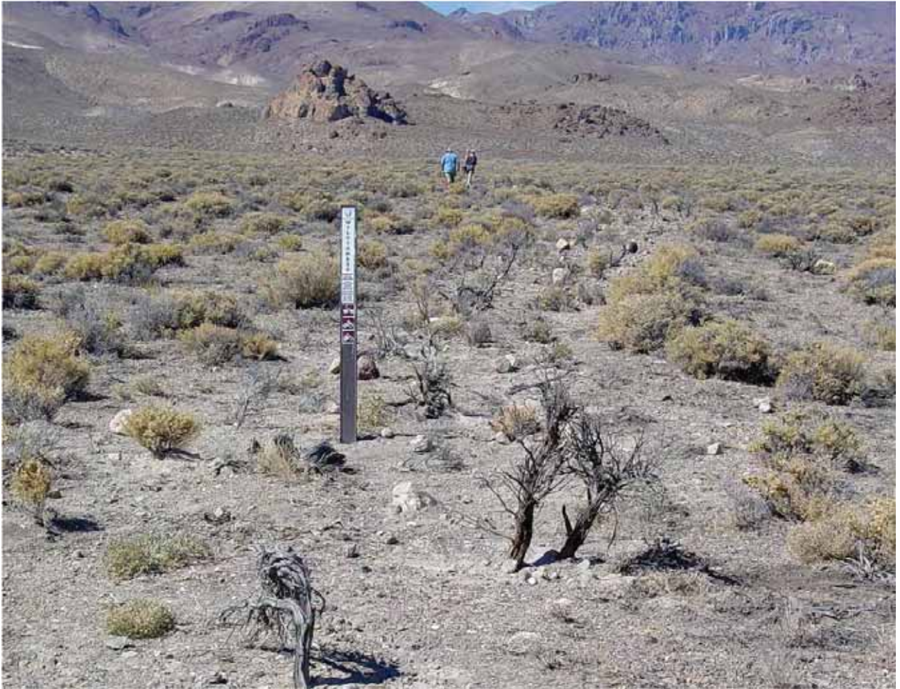
Vertical mulch in an abandoned roadway. (Credit: BLM.)
