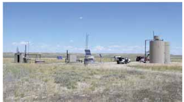
These grouped structures have been painted the same color to reduce visual contrasts with each other and with the surrounding vegetation. (Credit: BLM.)
