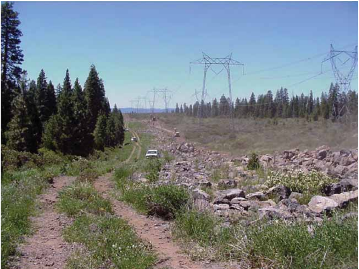
A two-track road built to provide access to a transmission ROW. (Credit: USDA Forest Service.)
