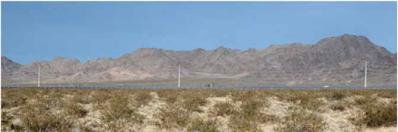
The power conversion units (inverters) at this thin-film PV facility were painted to match the vegetative background, greatly reducing the color contrast, and are difficult to see. Note however, how conspicuous the white monopole transmission towers are against the mountain backdrop. (Credit: Robert Sullivan, Argonne National Laboratory.)
