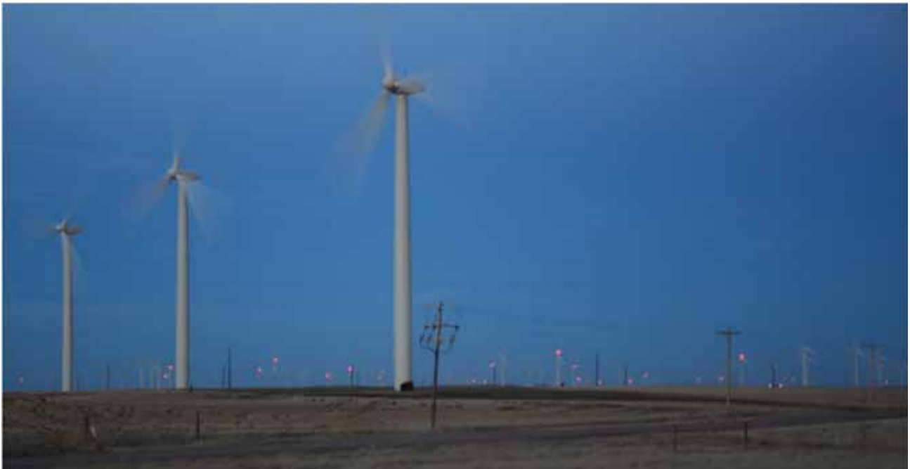
FAA-required hazard navigation lighting presents a major unavoidable source of night-sky impacts from utility-scale wind facilities. (Cedar Creek I Wind Farm, near Grover, Colorado. Credit: Robert Sullivan, Argonne National Laboratory.)
