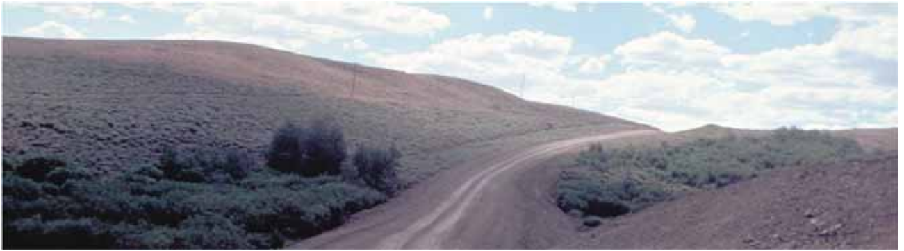
This road follows natural contours, reducing the need for cut and fill. (Credit: BLM)
