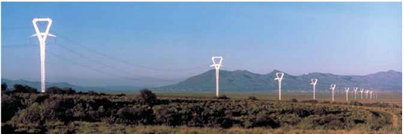
Glare from untreated galvanized guyed lattice transmission towers in low-angle sunlight. (Credit: BLM.)
