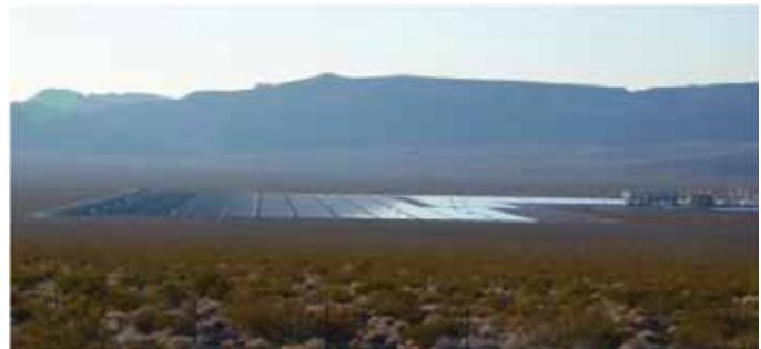
The polished surfaces of black photovoltaic solar panels are highly reflective. (Copper Mountain Solar Facility, near Boulder City, Nevada. Credit: Robert Sullivan, Argonne National Laboratory.)
