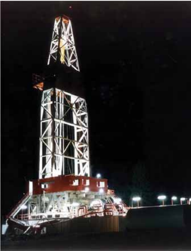
Geothermal drilling rig at night. (Long Valley Exploratory Well near Mammoth Lakes, California. Credit: Sandia National Laboratories.)
