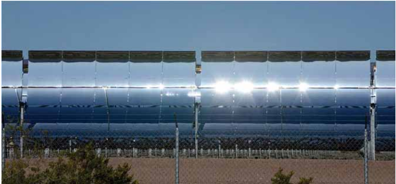
Close-up photo of parabolic trough mirrors showing glare sources. (Nevada Solar One near Boulder City, Nevada. Credit: Robert Sullivan, Argonne National Laboratory.)
