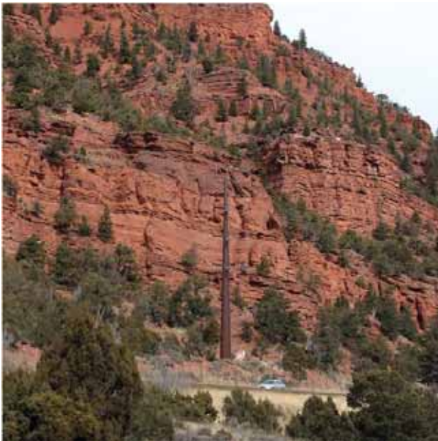
COR-TEN monopole in a high-relief landscape with minimal vegetation, and where the predominant natural color is red. (Credit: John McCarty, BLM.)
