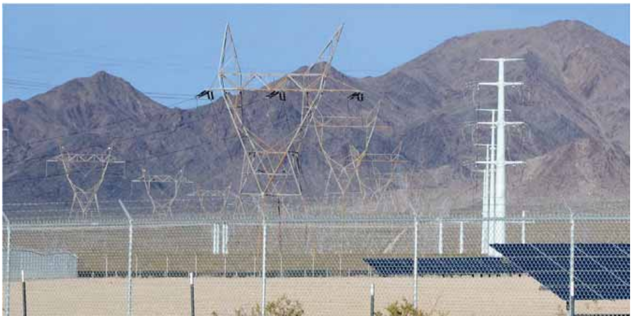
Lattice and monopole towers near solar facility. Lattice towers are generally less visible than monopoles against landscape backdrops. (Credit: Robert Sullivan, Argonne National Laboratory.)
