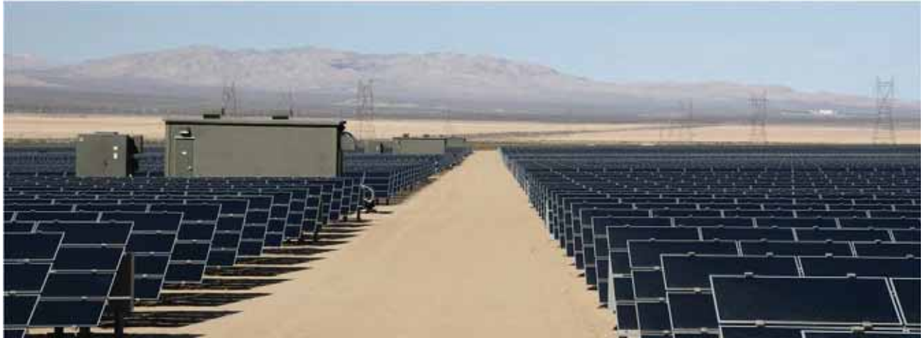
A well-maintained solar facility. (Credit: Robert Sullivan, Argonne National Laboratory.)
