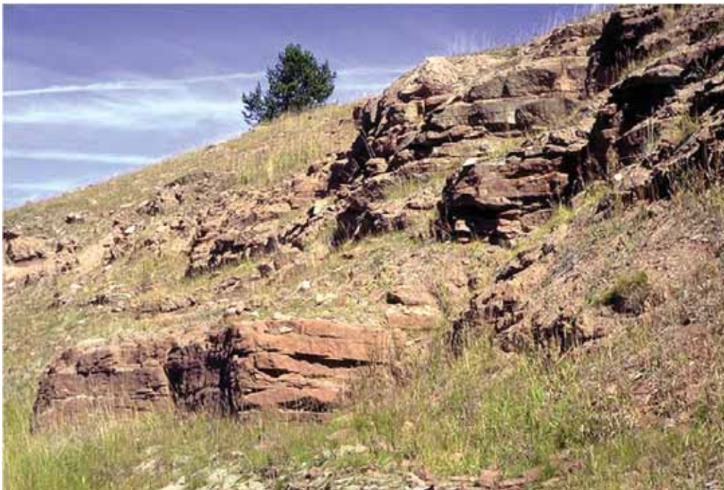
After revegetation, a properly shaped and sculpted rock cut blends in well with the surrounding landscape. (Credit: BLM.)
