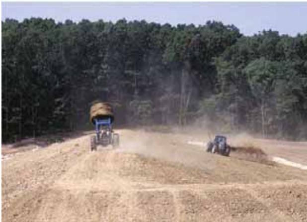
Mulch application. (Credit: Natural Resources Conservation Service.)
