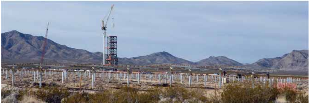
The Ivanpah Solar Energy Generating System, a CSP power tower facility currently under construction in the Ivanpah Valley in California, will utilize dry-cooling technology. (Credit: Robert Sullivan, Argonne National Laboratory.)
