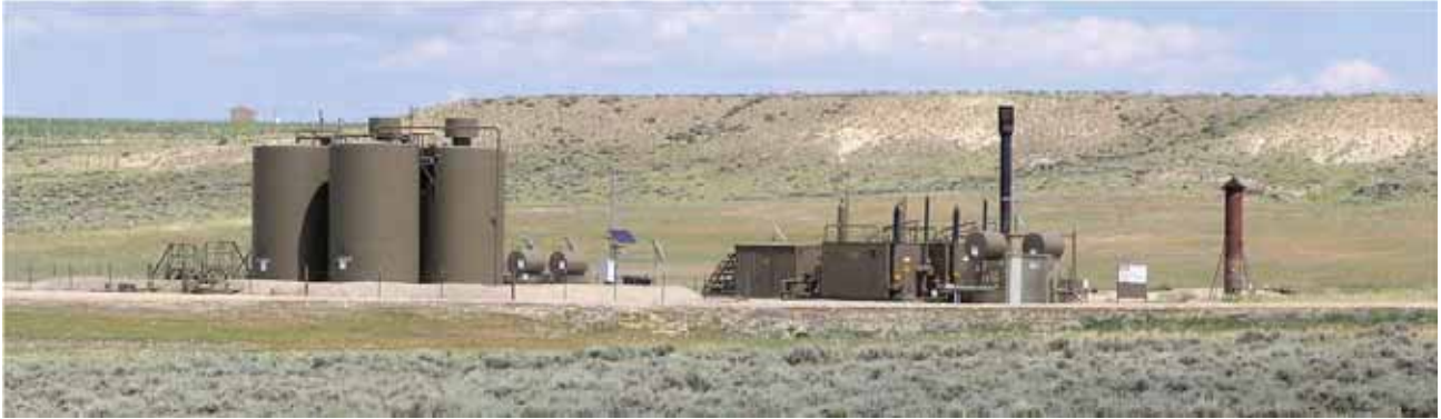
These structures have been painted the same color to reduce visual contrasts with each other and with the surrounding landscape. (Credit: BLM.)
