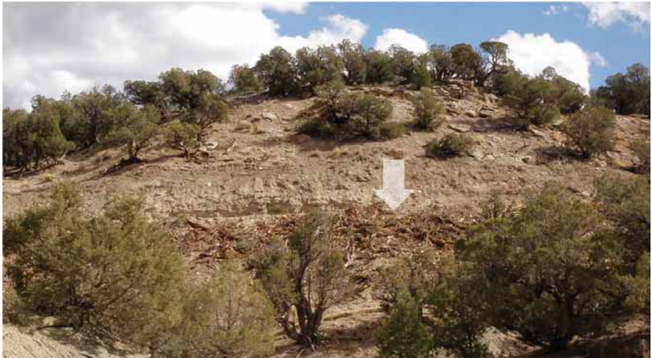
Slash used to stabilize slope below a road cut. (Credit: BLM.)
