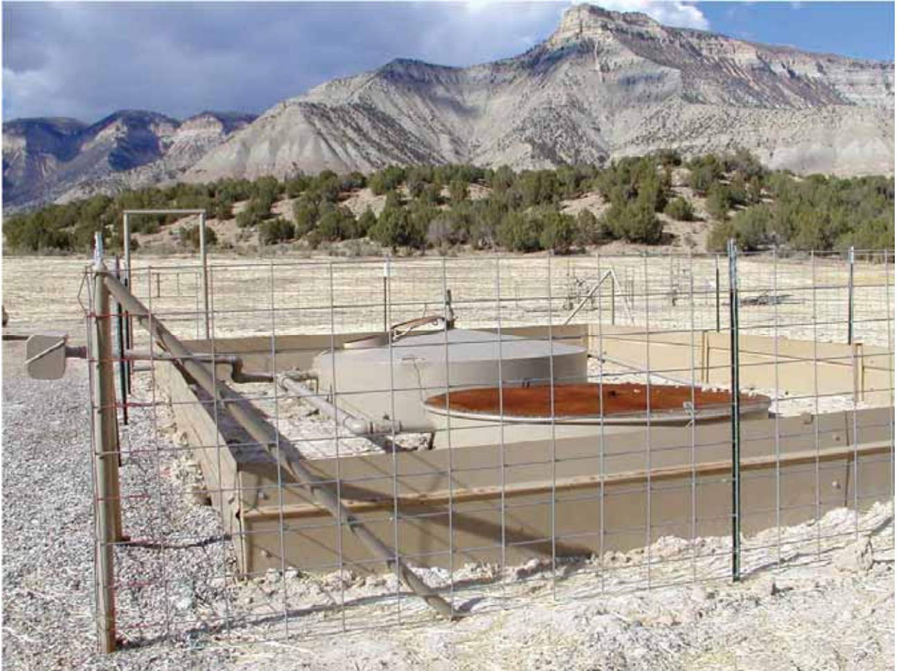
Partially buried tanks. (Credit: John McCarty, BLM.)
