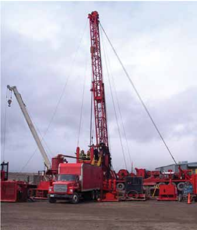
Geothermal drilling rig. (Credit: Idaho Department of Water Resources.)
