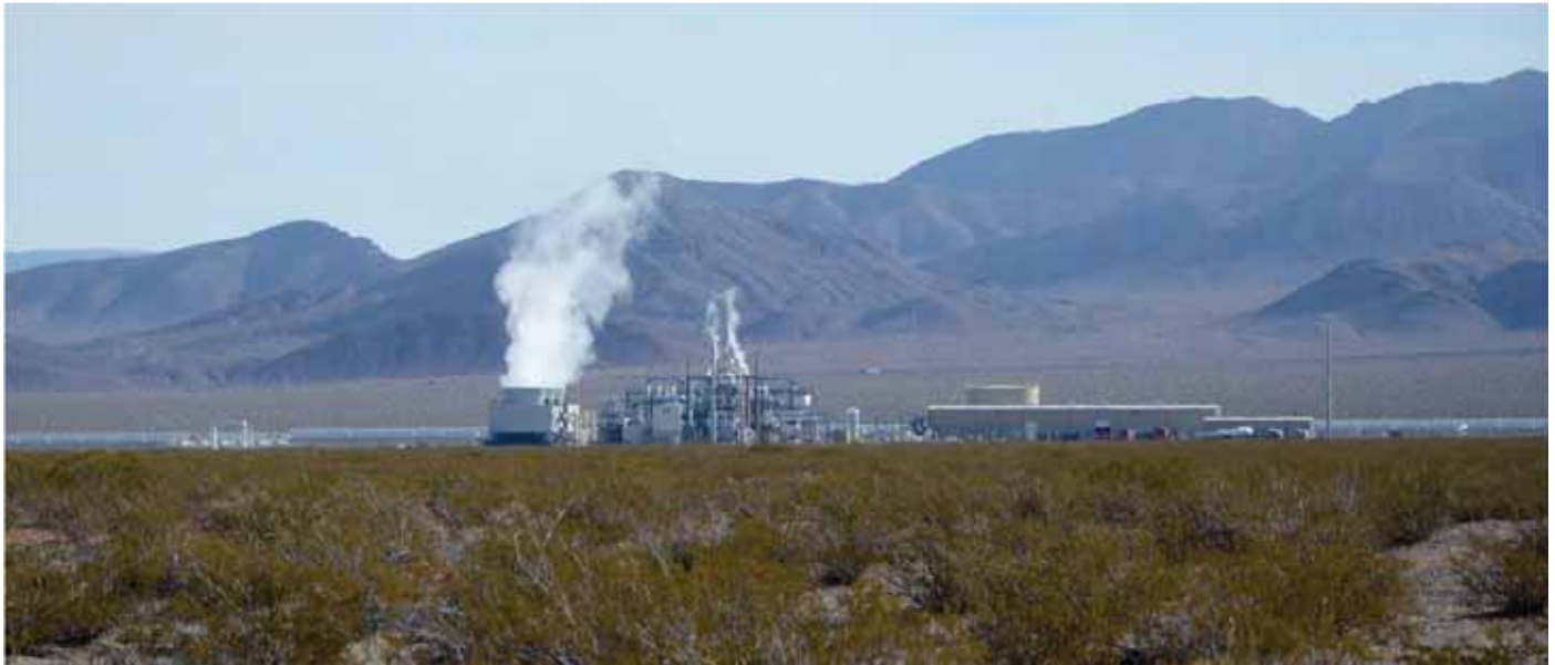
Ancillary structures at a parabolic trough facility, including cooling tower, steam turbine generator, and equipment shed. Note prominent plume. (Nevada Solar One near Boulder City, Nevada. Credit: Robert Sullivan, Argonne National Laboratory.)
