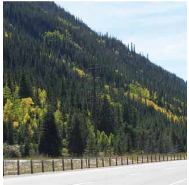
Color-treated monopole towers blend in well with the surrounding landscape, resulting in substantially lower visual contrast. (Credit: BLM.)
