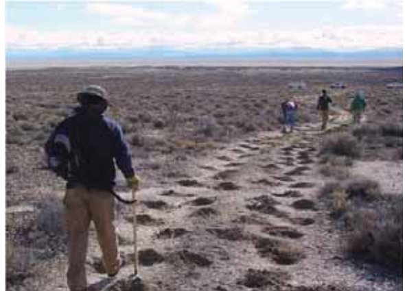
Pitting an abandoned roadway. (Credit: BLM.)
