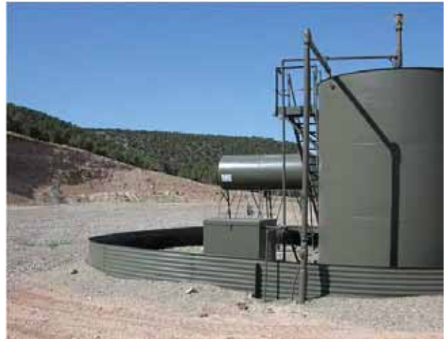
This structure has been painted with a BLM standard environmental color to reduce visual contrasts with the surrounding vegetation. (Credit: BLM.)
