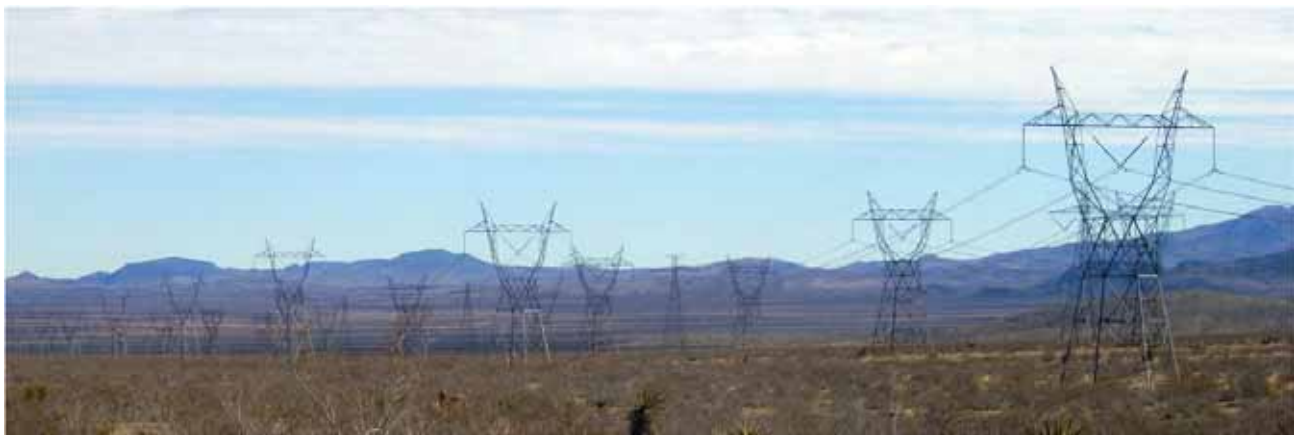
Collocation of transmission lines generally reduces overall visual impacts. (Credit: BLM.)
