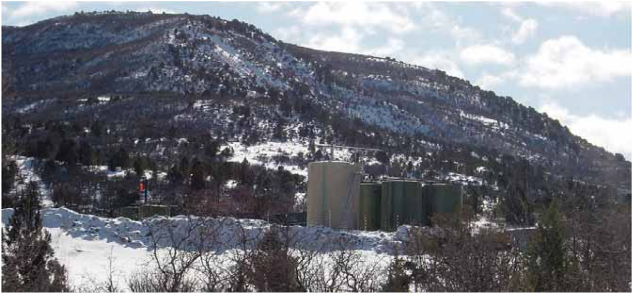
Tanks painted with two BLM standard environmental colors. The darker color is a better match for this landscape. (Credit: BLM.)
