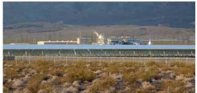
The power block, collector array, and buildings of this solar parabolic trough facility introduce a variety of non-natural textures to this landscape. (Nevada Solar One near Boulder City, Nevada. Credit: Robert Sullivan, Argonne National Laboratory.)
