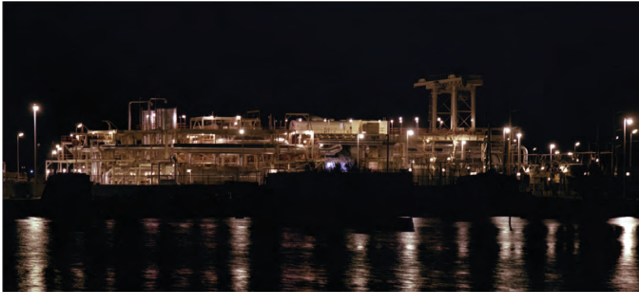
Nighttime shot of a geothermal power plant located near El Centro, California. Better lighting practices could substantially reduce light pollution from this facility. (Credit: Warren Gretz, NREL.)
