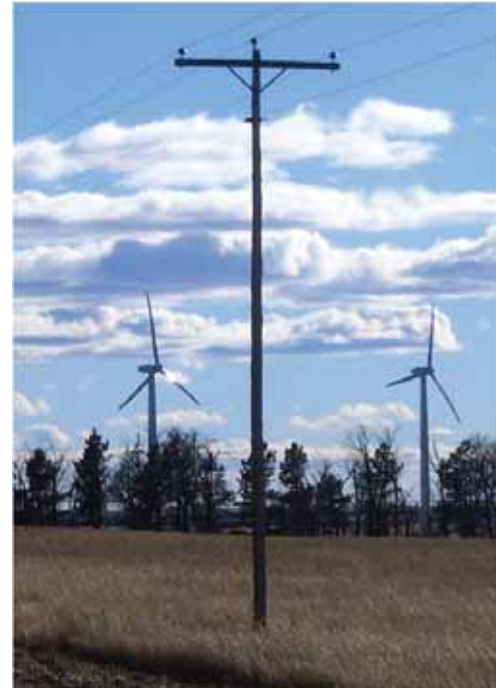
Blade glinting near hub of turbine at left. These bright flashes from sunlight falling on the reflective surface of the blade have been observed at distances exceeding 15 mi, and can increase turbine visibility considerably. (Cedar Creek 1 Wind Farm, near Grover, Colorado. Credit: Robert Sullivan, Argonne National Laboratory.)
