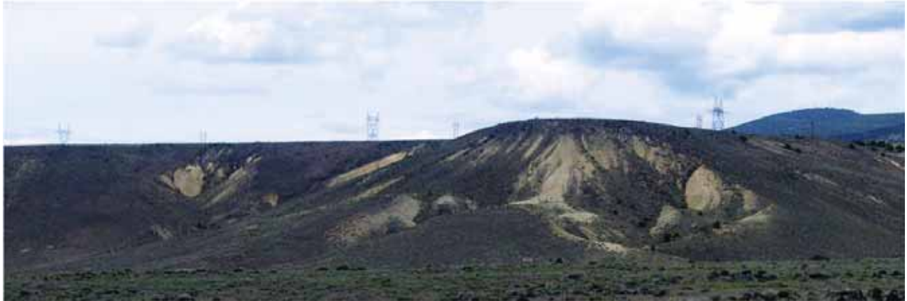
Skylining of transmission lines makes them conspicuously visible against the sky backdrop. (Credit: BLM.)
