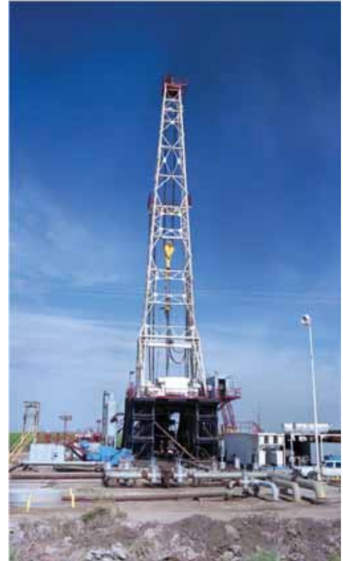
Geothermal production well drilling. (Imperial Valley, California. Credit: Warren Gretz, NREL.)
