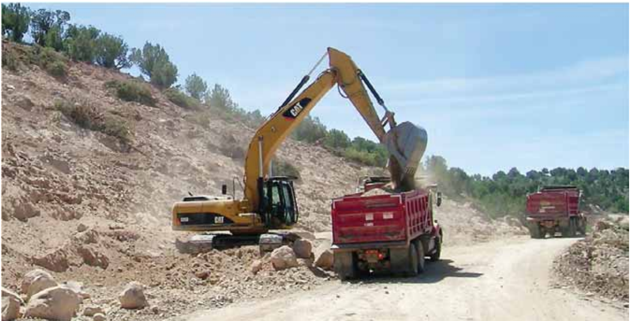
Excess fill being removed for offsite storage. (Credit: BLM.)
