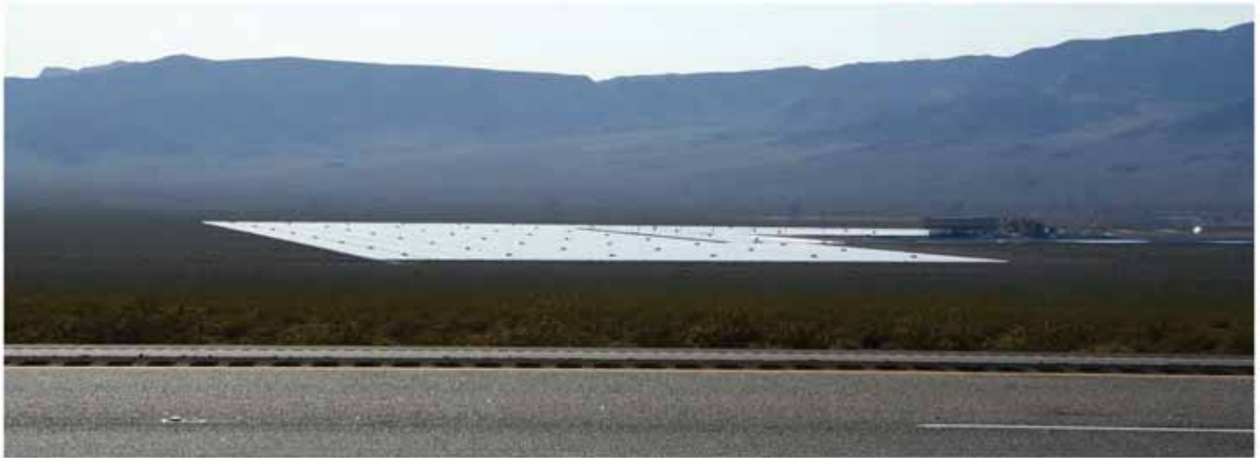
Apparent color changes with differing sun angle and viewing geometry at thin-film PV facility. Note contrasting color of regularly spaced inverter boxes among the panels in the collector array. (Copper Mountain Solar Facility, near Boulder City, Nevada. Credit: Robert Sullivan, Argonne National Laboratory.)
