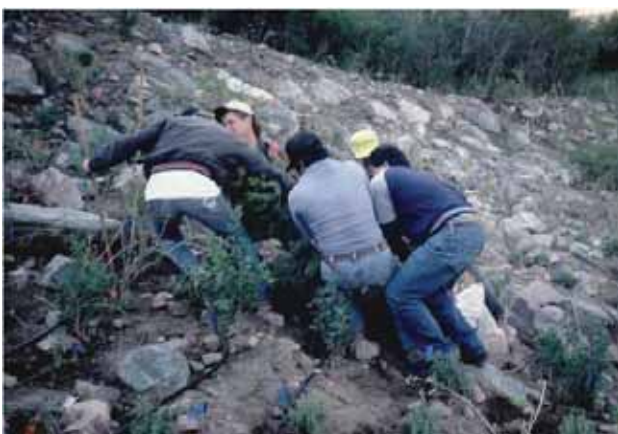
Planting a conifer in a planting pocket. (Credit: John McCarty, Colorado Department of Transportation.)
