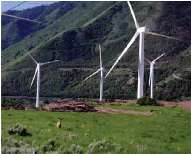
Non-linear turbine configurations are better suited to rolling terrain. (Spanish Fork Wind Farm, Utah. Credit: NREL.)
