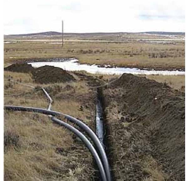
Burying a small pipeline. (Credit: BLM.)
