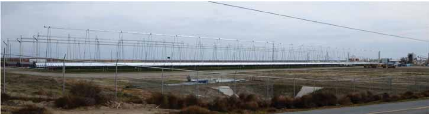
Close-up photo of Kimberlina CLFR facility near Bakersfield, California. Mirrors are the white band running left to right across the photo. The receiver tubes are held well above the mirrors. Ancillary buildings, including STG, are at far right. (Credit: Robert Sullivan, Argonne National Laboratory.)
