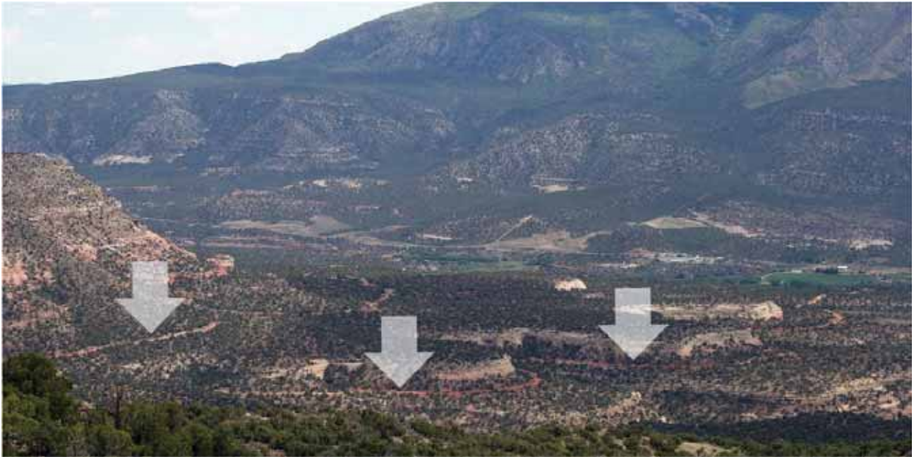
This road follows the undulating contours of the landform, making it less visually prominent. (Credit: John McCarty, BLM.)
