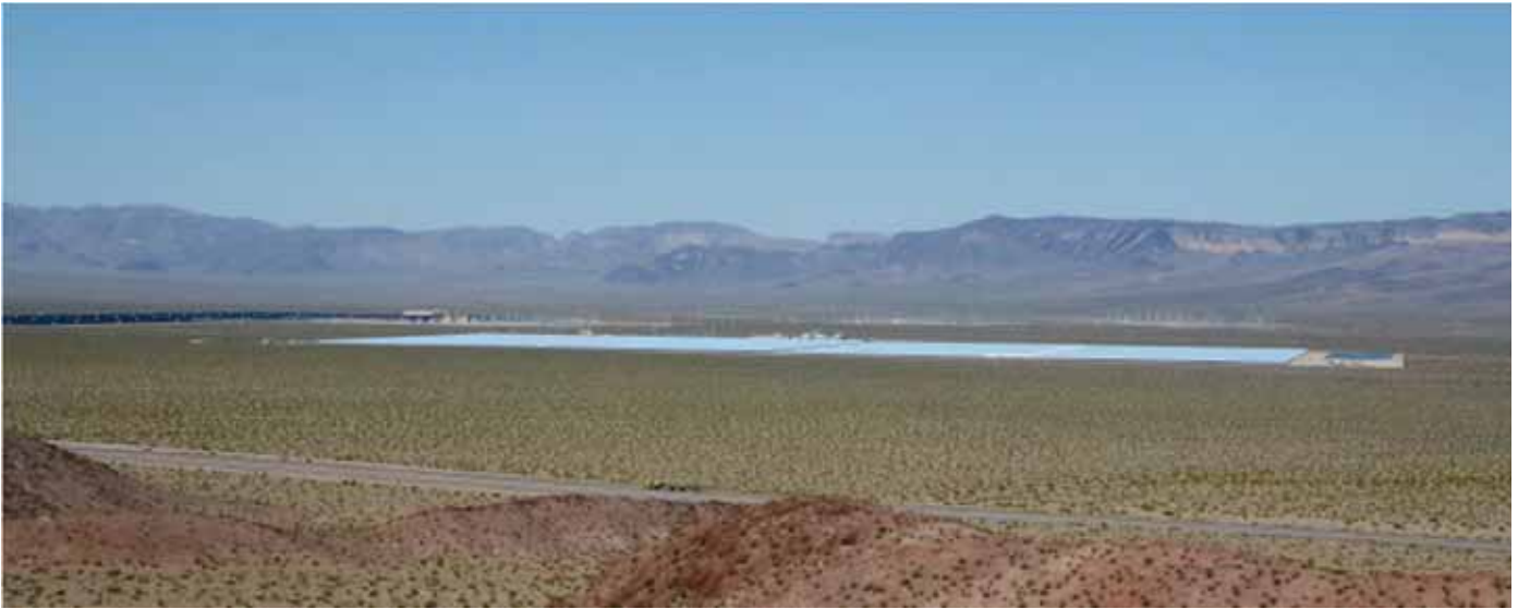
Operating solar facilities near Boulder City, Nevada: Nevada Solar One parabolic trough facility at center and right; Copper Mountain thin-film PV facility at left. The large building adjacent to the Copper Mountain facility at left is a natural gas power plant. A large substation is visible behind the facilities. (Credit: Robert Sullivan, Argonne National Laboratory.)
