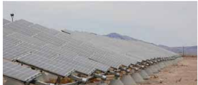
Flat plate PV: Crystalline silicon PV panels on tilted single-axis trackers. (Nellis Air Force Base, Nevada. Credit: Robert Sullivan, Argonne National Laboratory.)
