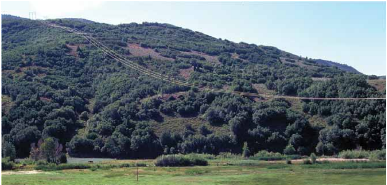
The clearings for transmission towers in this photo were shaped to blend in well with the naturally occurring clearings on the hillside. Although the conductors are plainly visible in this lighting, the dark tower color makes the towers difficult to see against the dark colors and varied textures of the vegetation. (Credit: BLM.)
