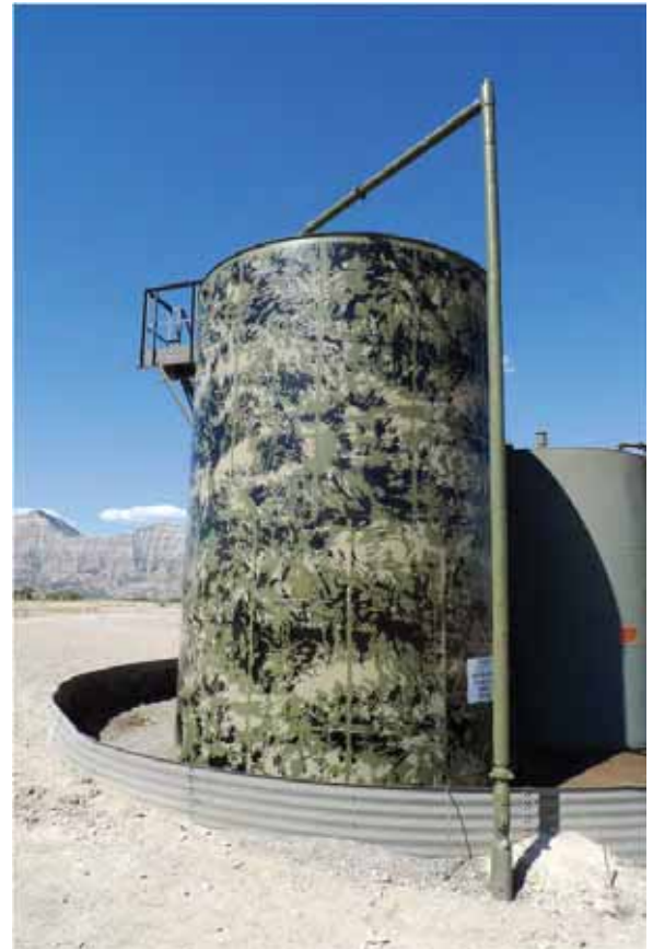
Color camouflage application on tank. (Credit: BLM.)
