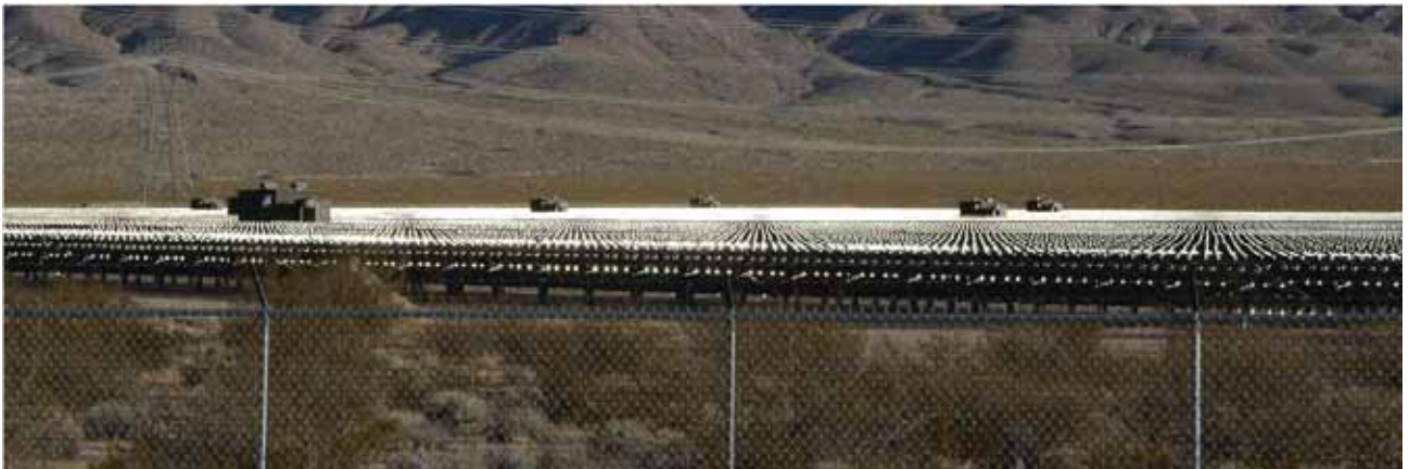
Reflected light from surfaces of just a few square inches of uncoated metal repeated on thousands of solar panel mounting structures creates an arresting high-contrast visual display. (Credit: Robert Sullivan, Argonne National Laboratory.)
