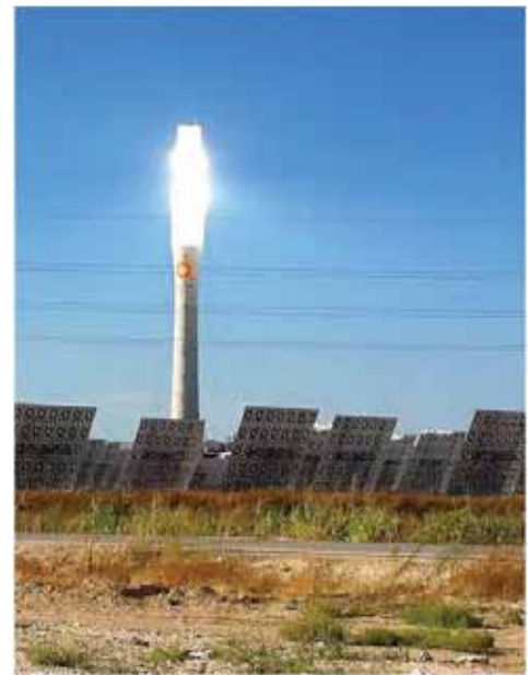
Offsite glare from 20-MW power tower facility. (Torresol Gemasolar facility near Seville, Spain. Credit: Robert Sullivan, Argonne National Laboratory.)
