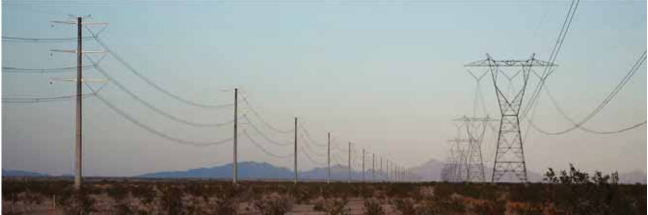
Untreated galvanized monopole transmission towers (left) and lattice towers (right). Note monopole crossbar reflectivity even in distant background, and greater visual weight of monopoles beyond the immediate foreground. (Credit: Robert Sullivan, Argonne National Laboratory.)
