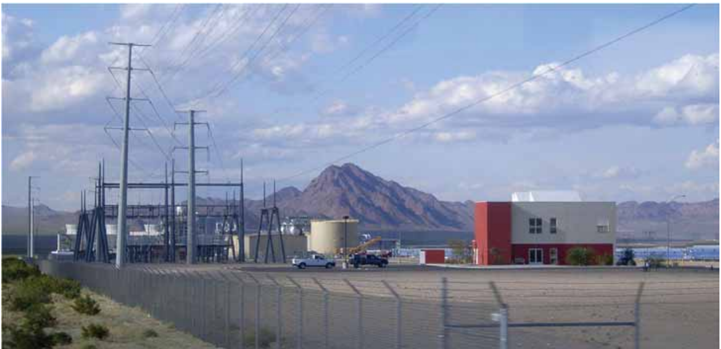
Ancillary structures at a parabolic trough facility, including substation, administration building, equipment shed, and HTF tank. Steam turbine generator and cooling tower visible behind substation. Solar collector array visible at far right. (Nevada Solar One near Boulder City, Nevada. Credit: Robert Sullivan, Argonne National Laboratory.)
