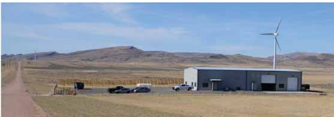
Wind energy facility control building, fences, and parking area. (Dunlap Ranch Wind Energy Project near Medicine Bow, Wyoming. Credit: Robert Sullivan, Argonne National Laboratory.)
