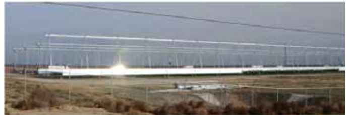
Glare from reflected sunlight on a solar Compact Linear Fresnel Reflector mirror. (Kimberlina Solar Thermal Energy Plant near Bakersfield, California. Credit: Robert Sullivan, Argonne National Laboratory.)
