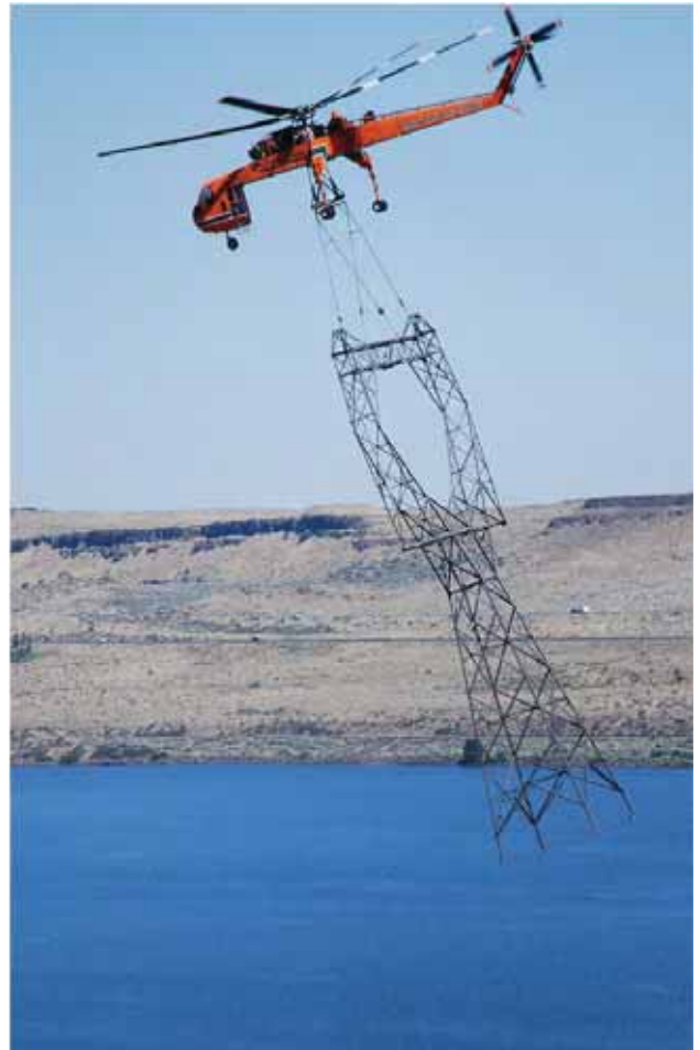
Helicopter transporting pre-assembled transmission tower. (Credit: Bonneville Power Administration.)
