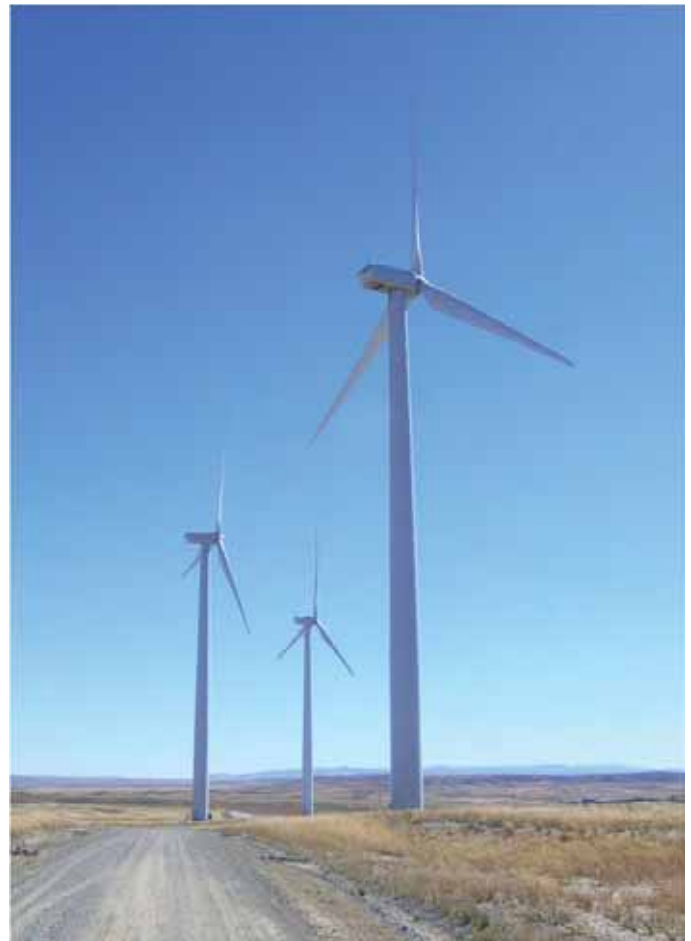
Wind turbines create strong vertical line contrasts in flat landscapes with strong horizon lines. (Dunlap Ranch Wind Energy Project near Medicine Bow, Wyoming. Credit: Robert Sullivan, Argonne National Laboratory.)
