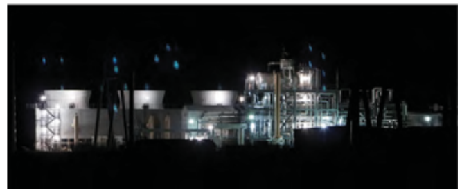
Power block of operating solar parabolic trough facility. (Nevada Solar One near Boulder City, Nevada. Credit: Marc Sanchez, BLM.)
