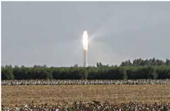
Glare and reflections from airborne dust particles at Torresol Gemmasolar 20-MW power tower facility near Seville, Spain. (Credit: Robert Sullivan, Argonne National Laboratory.)
