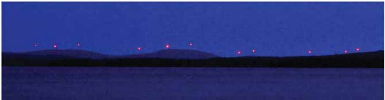
Conventional hazard navigation lights atop wind turbines. (Credit: Terry DeWan, Terrence J. DeWan & Associates.)
