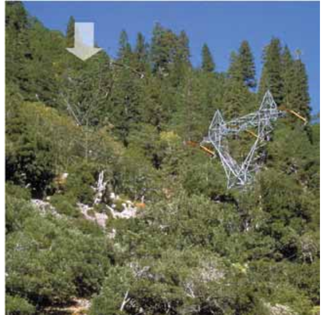
The color-treated lattice tower to the upper left of the untreated tower blends in very well with the surrounding landscape, and could easily be missed by a casual viewer. (Credit: John McCarty, BLM.)
