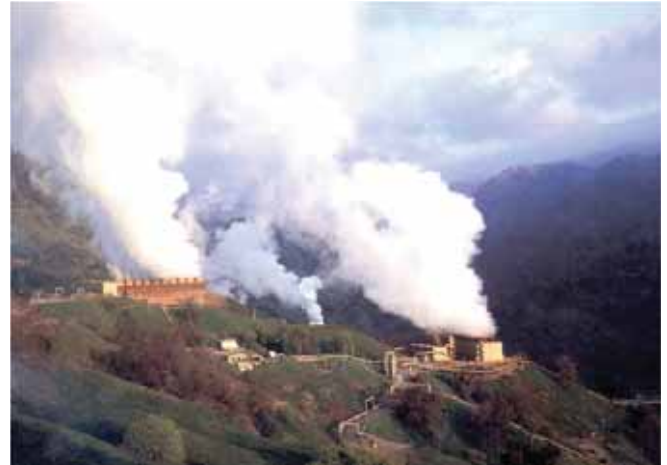
Steam plumes rise from cooling towers at a dry steam plant. (Geysers facility near Calistoga, California. Credit: U.S. Geological Survey.)
