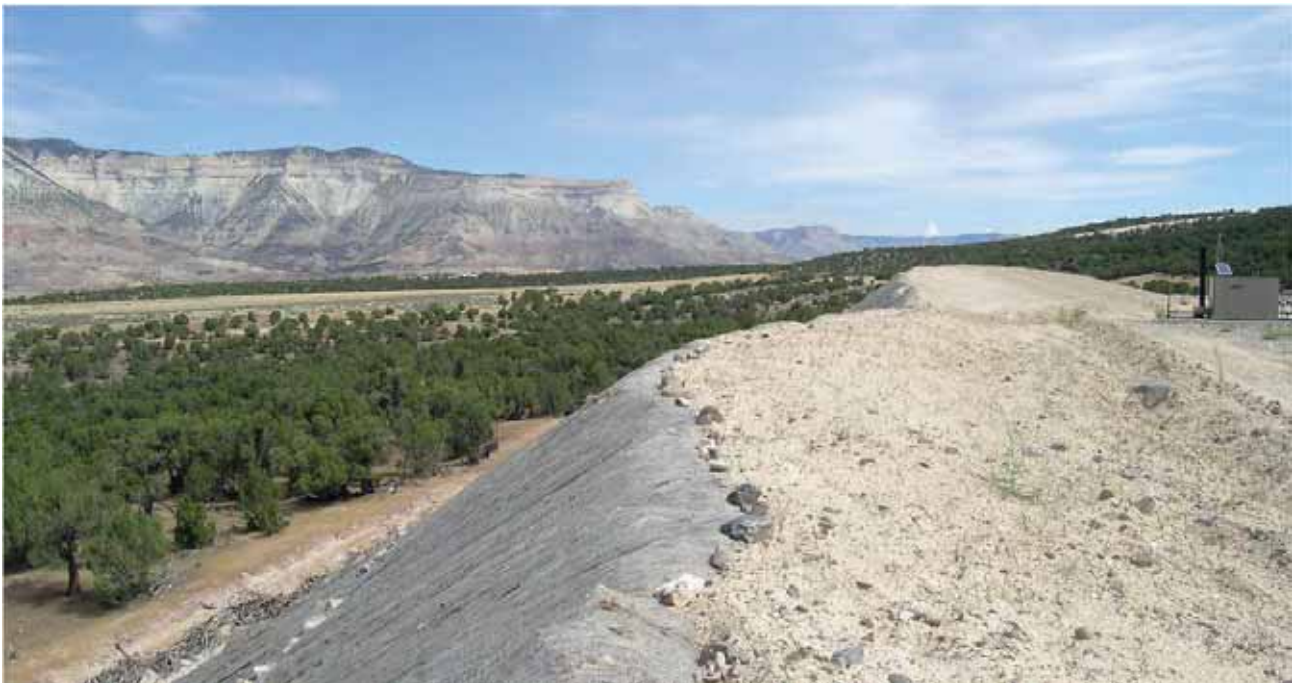
A stabilized and seeded slope. (Credit: BLM.)
