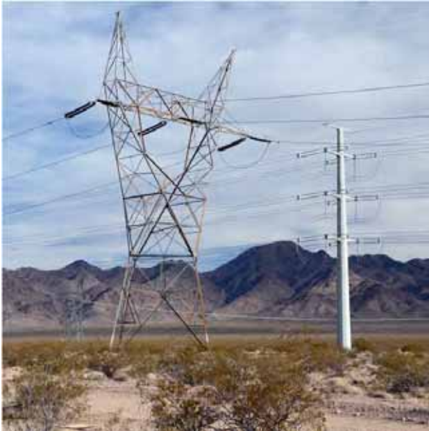
Weathered lattice tower and white monopole. An additional lattice tower is visible in the background to the left of the large lattice tower. (Credit: Robert Sullivan, Argonne National Laboratory.)
