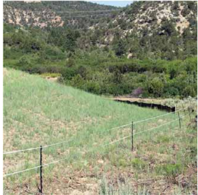
An example of erosion control good practices: the reseeded area is fenced off and the silt fence left in place until vegetation is re-established. (Credit: BLM.)
