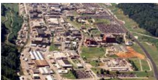
Y-12 National Security Complex
