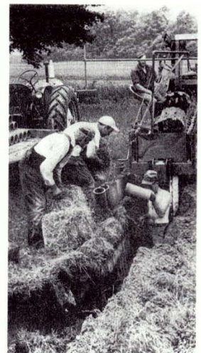
Drainage tile operation, circa 1940’s. Tiles provide a conduit for moving water from a wetland. (Photograph courtesy of U.S. Department of Agriculture.)
