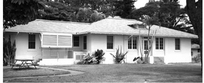
Commanding Officer's House (Facility A) at the Radio Transmitter Facility Lualualei. Constructed in 1937. (Source: Mason Architects, Inc.)
