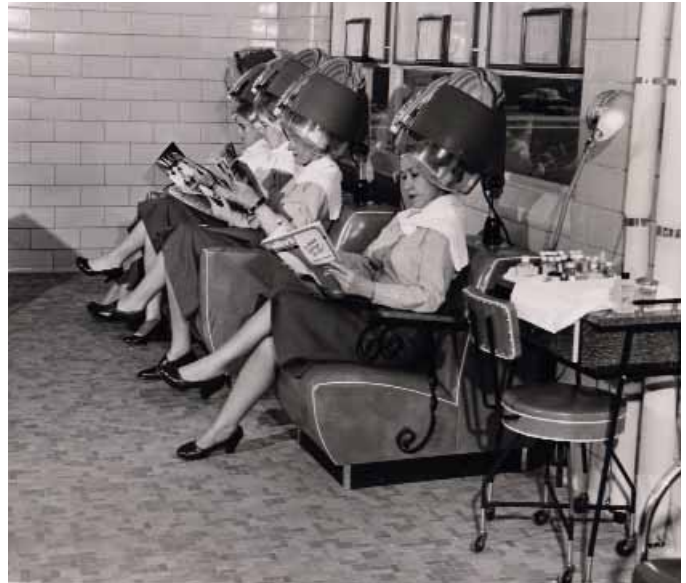
Fort McClellan, WAC Center Beauty Shop, 1954 (US Army Women's Museum, File: UA WAC School-Facilities/Buildings/Grounds VI-A-17).
