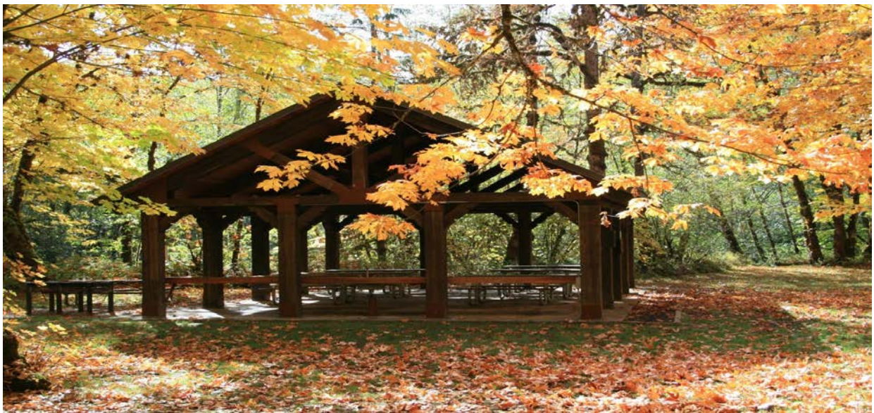
Rock Creek Pavilion
