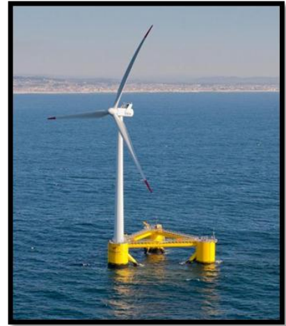
Floating Wind Turbine. Photo: Courtesy of Principle Power
