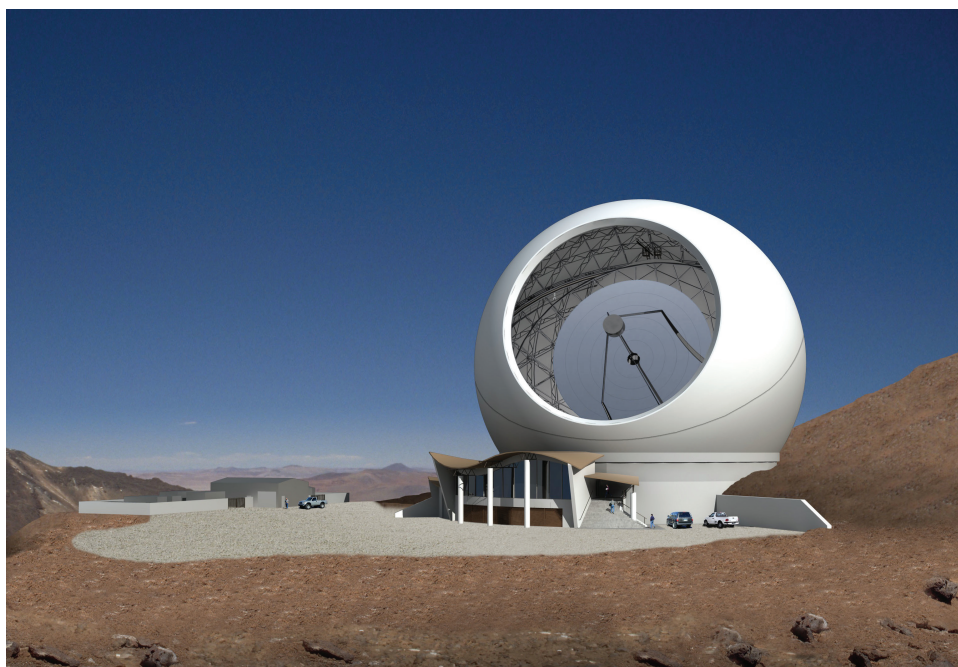
FIGURE 7.11 CCAT is a 25-meter telescope located at 18,500 feet elevation close to ALMA in Chile. The mirror surface has active control. CCAT will operate from 0.3 to 1.4 millimeters (with a goal of 0.2 to 3.5 mm) with a 10- to 20-arcminute field of view and diffraction-limited angular resolution of 10 \times (wavelength in millimeters) arcsecond. Highly sensitive bolometer arrays with more than 10,000 sensors using superconducting transition edge sensor technology are envisaged. The flux sensitivity is limited by source confusion to around 1 mJy. SOURCE: M3 Engineering/CCAT/Caltech.
