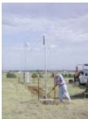
Installation of the OK-LMA
