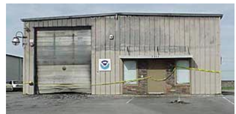
NSSL's equipment storage facility after the fire.
