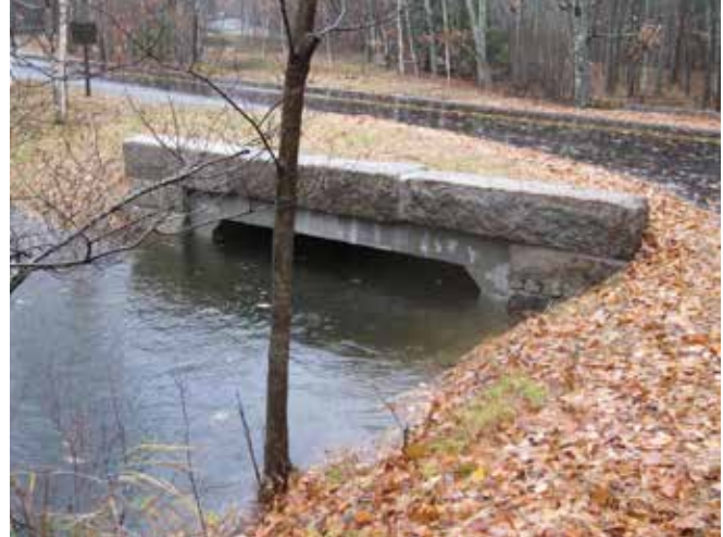
Headwall and culvert after rehabilitation at Sieur de Monts Spring site. Image credit: Rebecca Cole-Will.
