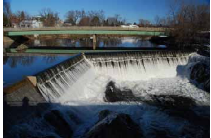
Figure 10. The Kendall Plant Dam at Enosburg Falls. Photo by Ken Secor.
