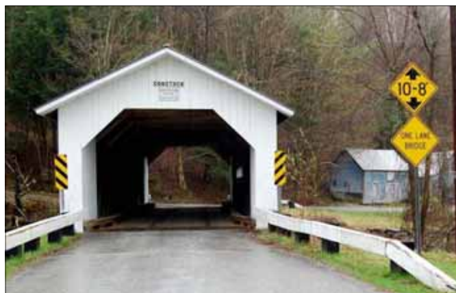
Figure 50. Comstock Bridge, Montgomery, VT. Photo by Ken Secor
