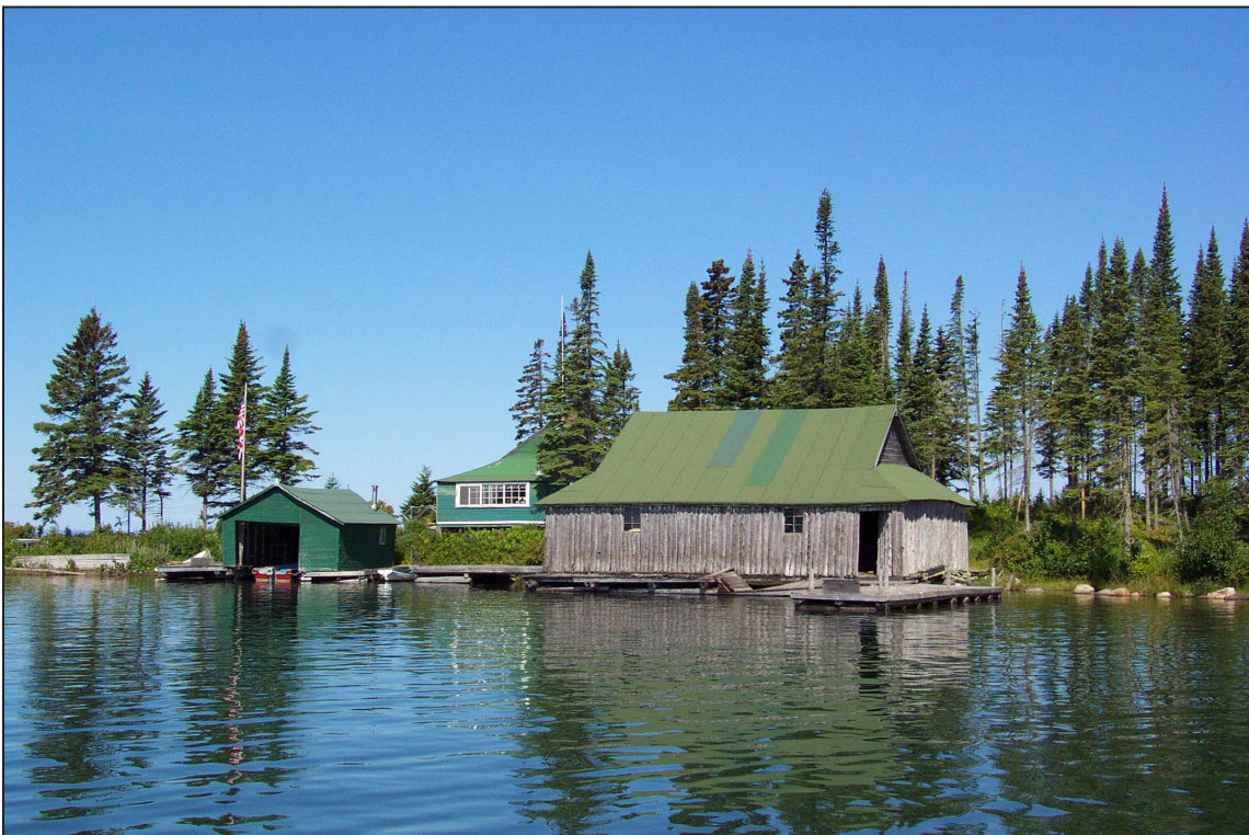
Historic Barnum cabin in Isle Royale National Park. Stronger and more frequent storms (e.g., ice storms and wildfires) may adversely impact historic structures such as these. NPS photo.
