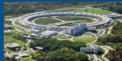
Aerial view of the Advanced Photon Source at Argonne National Laboratory Photo courtesy of Argonne National Laboratory
