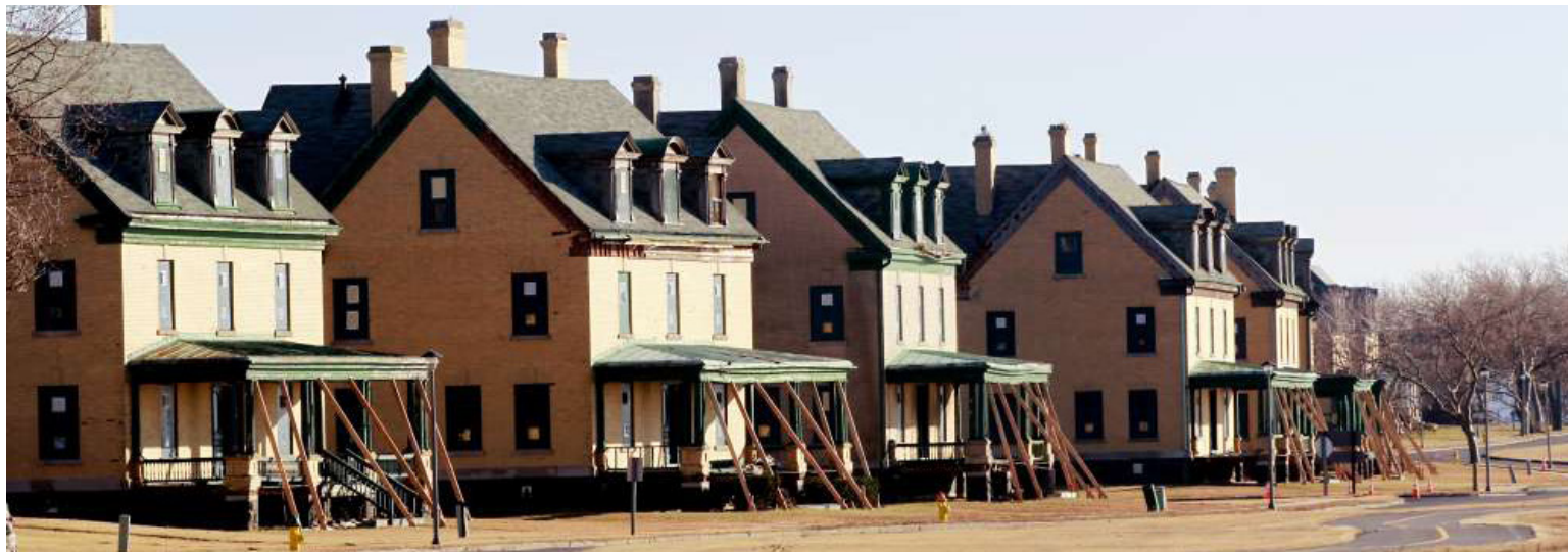
Buildings in Gateway National Recreation Area's Fort Hancock Historic Landmark District were devastated by Hurricane Sandy in 2012.
