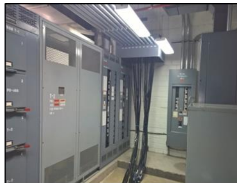
Spedding Hall—New 120/208V Electrical Distribution System (In-progress)
