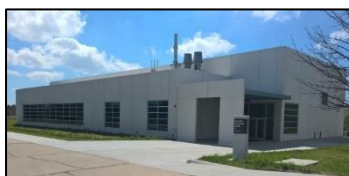
Sensitive Instrument Facility-SIF (2015)
