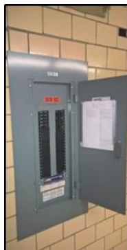
Spedding Hall—New 120/208V Electrical Distribution System (In-progress)
