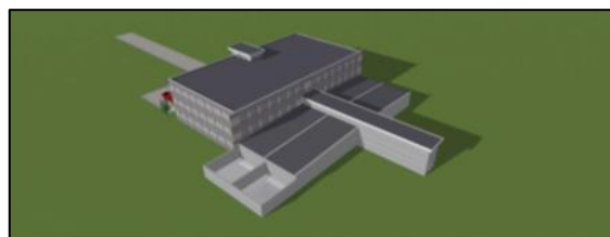
Scientific Computing Facility—Rear View—showing a long “spine” allows allowing for future expansion
