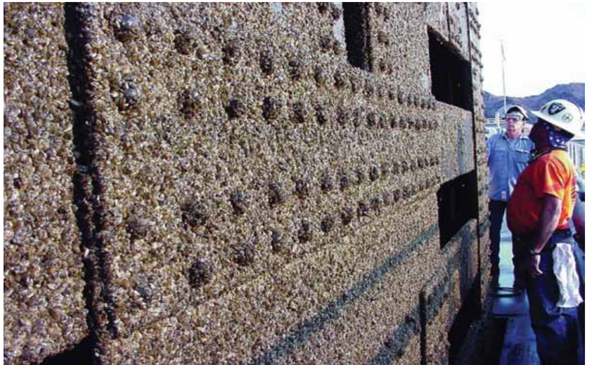
Quagga mussels encrust a penstock gate at Davis Dam on Lake Mohave, Arizona.
