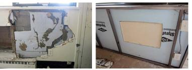
Existing condition of exterior wall insulation (left). Air sealing and insulating through-wall air-conditioning sleeve and exterior wall (right).
