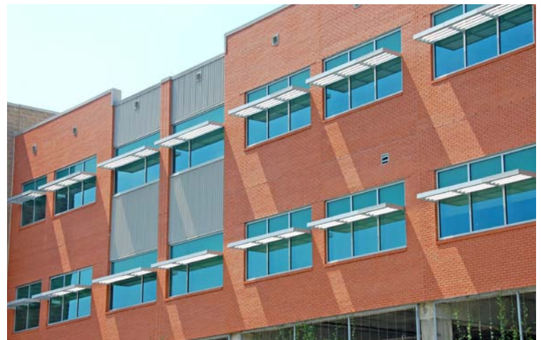
The majority of classrooms at Lake Area High School utilize daylighting thanks to the use of exterior shading and semi-transparent daylight glazing on the upper half of south-facing windows. Photo by Joe Ryan, NREL/PIX 19627
