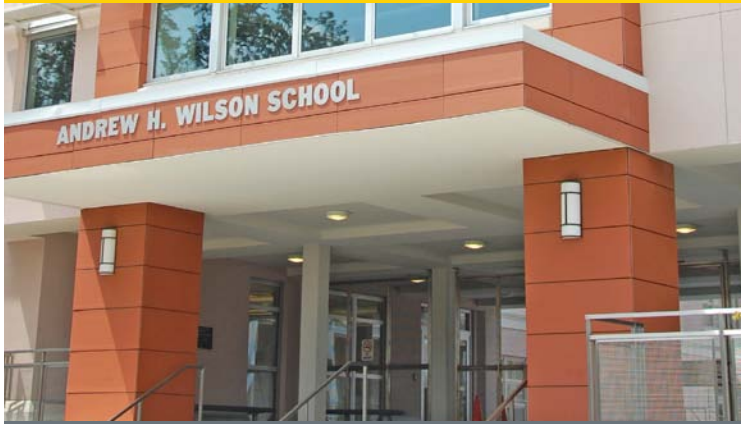
Andrew H. Wilson Elementary School, built in 1909, underwent a major renovation following Hurricane Katrina after suffering major flooding and wind damage. In addition to renovating the existing building, the school doubled its square footage and added both photovoltaic and solar hot water systems. Photo by Joe Ryan, NREL/PIX 19648
