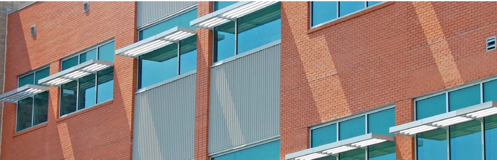
The majority of classrooms at Lake Area High School utilize daylighting thanks to the use of exterior shading and semi-transparent daylight glazing on the upper half of south-facing windows. Photo by Joe Ryan, NREL/PIX 19627
