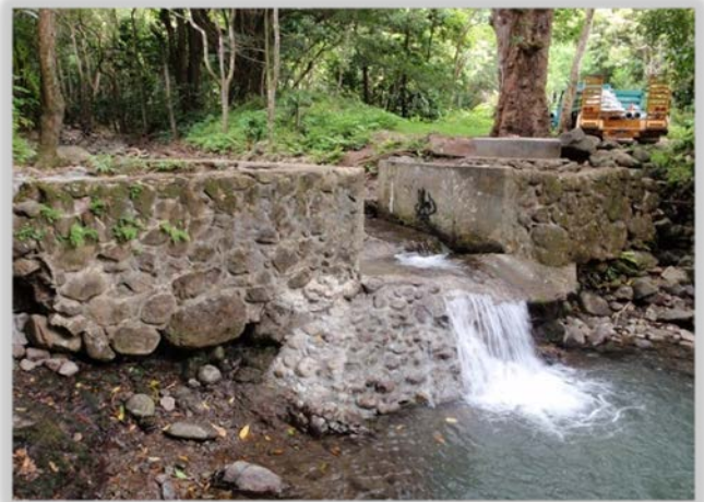
The modified instream structure provide a surface native species can ascend. Credit: Gordon Smith/USFWS
