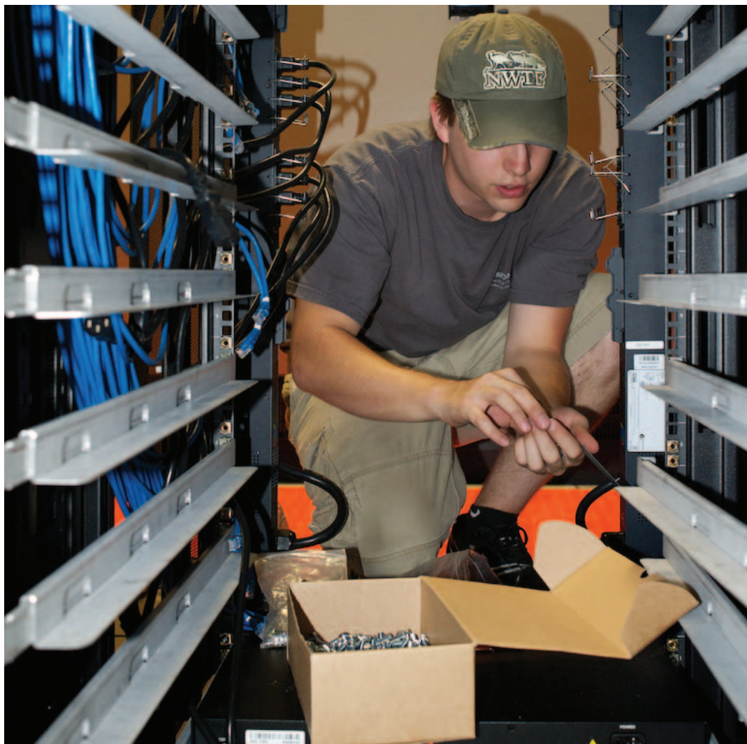
Installing tJet. Photo by Will von Dauster, ESRL.
