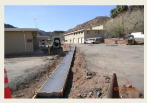
The contractor for the floating pump system mobilized on March 29, 2016. Excavation started to replace a section of pipe and valves.
