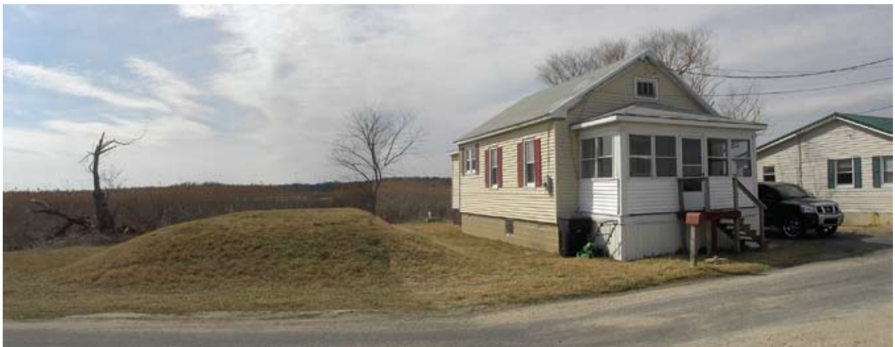
Figure 12.9 Mounds-based septic system next to house along the back side of Pickering Beach, Delaware (March 2009). [Photo source: ©James G. Titus, used with permission].
