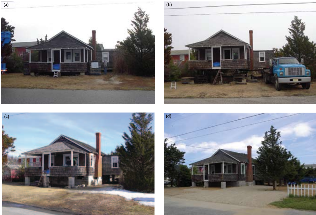
Figure 12.5 Elevating land and house (January through June 2005). (a) Initial elevation of house in Brant Beach, New Jersey. (b) Structural beams placed under house, which is lifted approximately 1.5 meters by hydraulic jack in blue truck. (c) Three course of cinder blocks added then house set down onto the blocks. (d) Soil and gravel brought in to elevate land surface. [Photo source: ©James G. Titus, used with permission].
