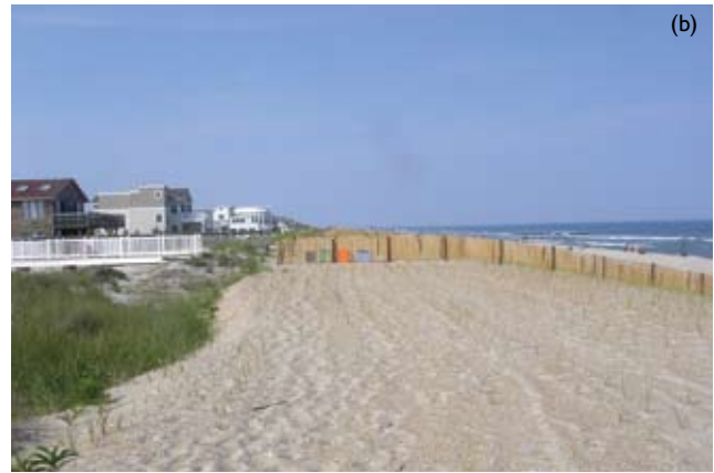
Figure 6.4 (a) A dike in Miami-Dade County, Florida (June 2005), and (b) a newly-created dune in Surf City, New Jersey (June 2007) [Photo source: ©James G. Titus, used with permission].
