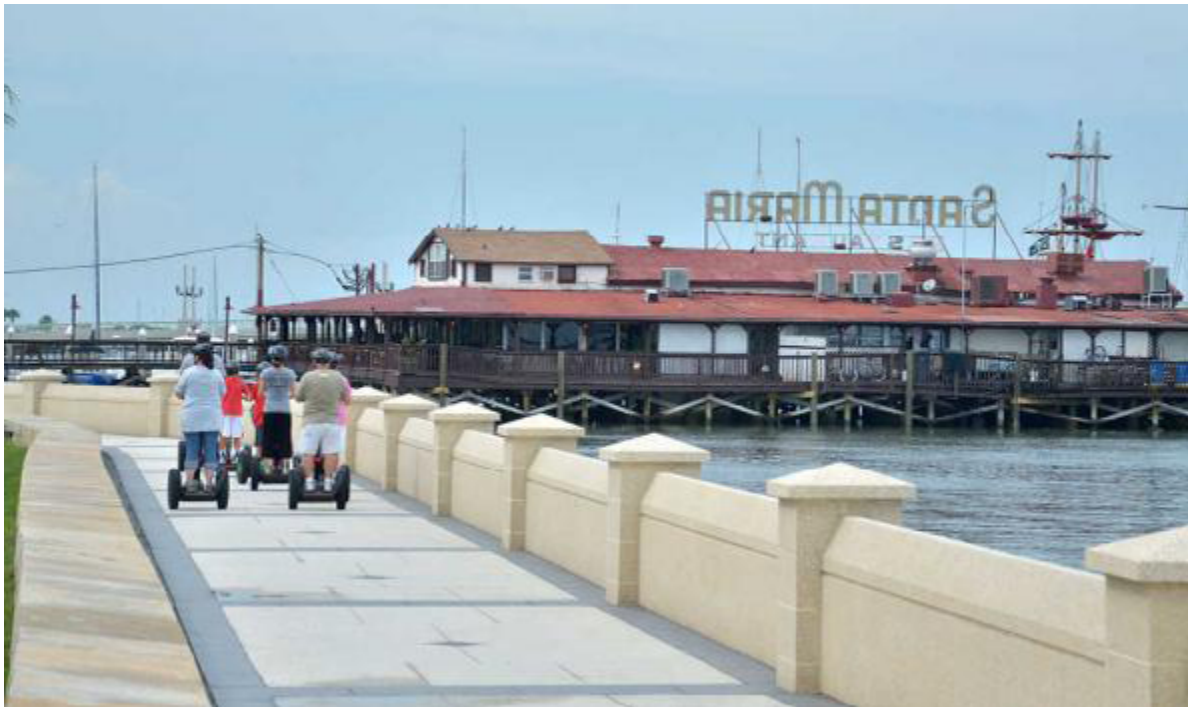
Figure 75. New seawall and preservation of historic seawall, St. Augustine. Source: http://staugustine.com/news/local-news/2014-07-09/visitors-locals-enjoying-new-seawall
