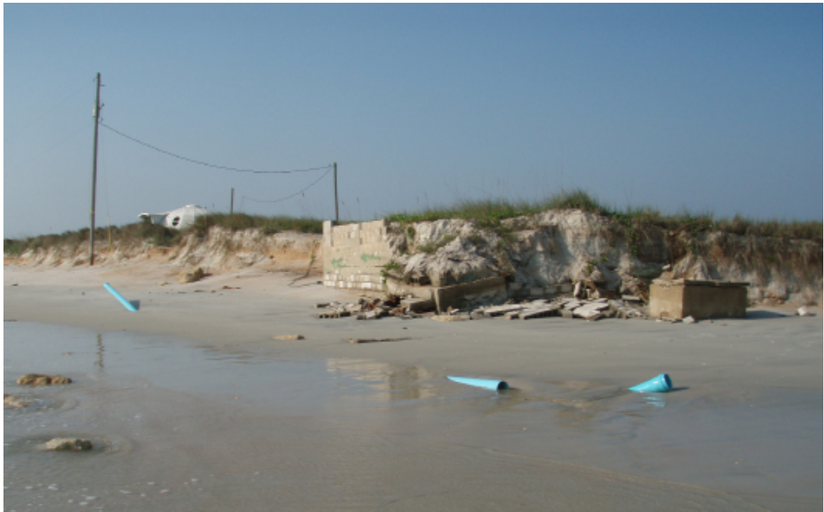
Figure 15. Remaining house foundation and septic tank. Source: Florida Sea Grant
