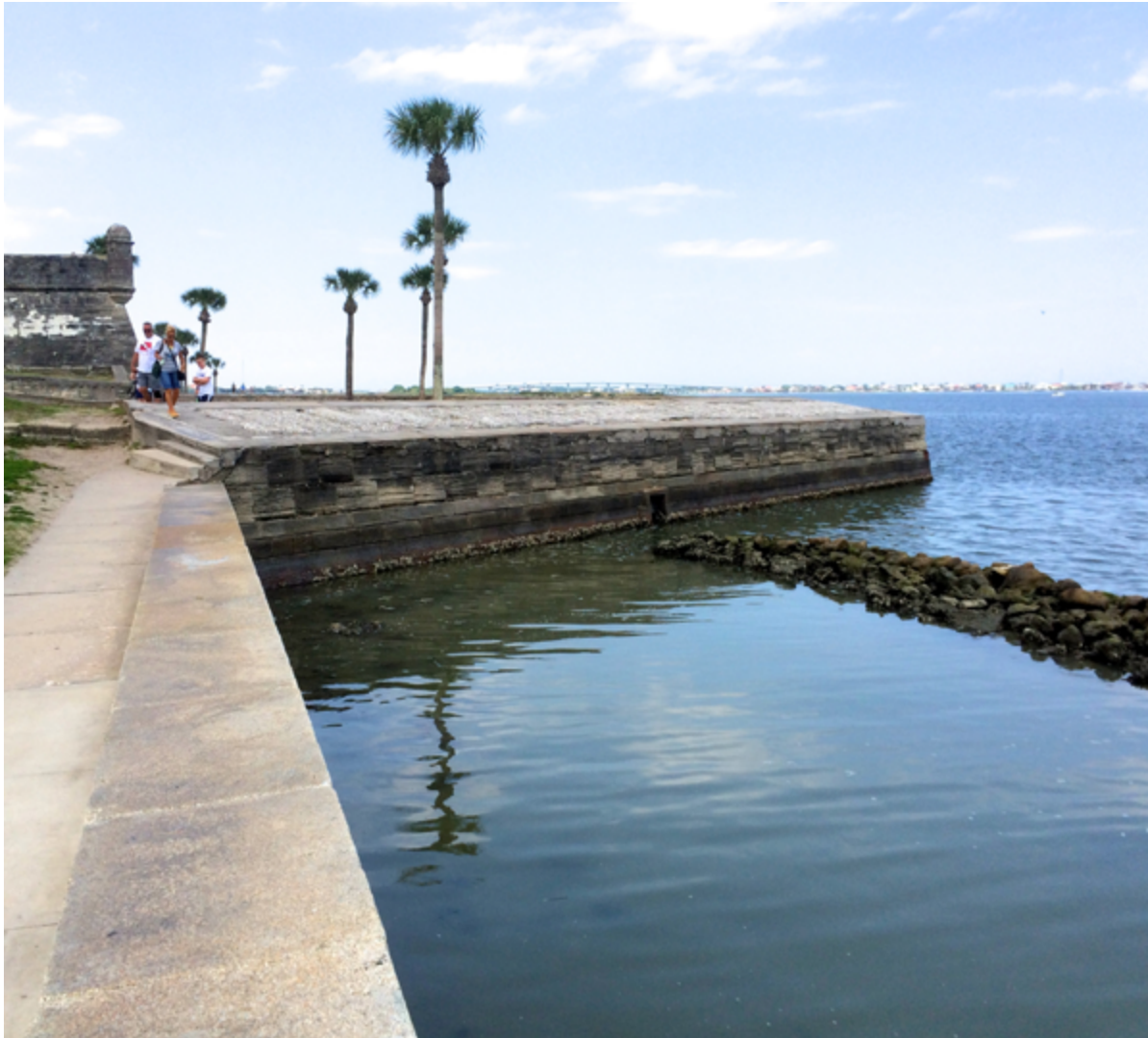
Figure 78. Living shoreline installed to protect the historic seawall at Castillo de San Marcos, St. Augustine
