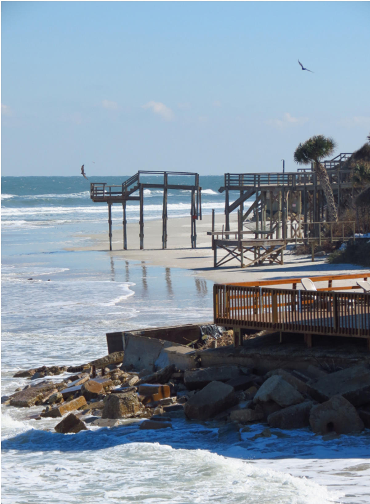
Erosion at Matanzas Inlet. Photo by Ed Siarkowicz Photographic Images, LLC
