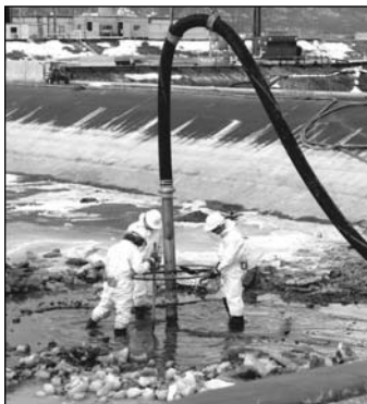
Pond sludge removal at Rocky Flats
