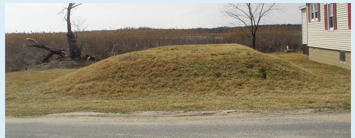
As sea level rises, the water table rises as well, which can prevent ordinary septic systems from working properly. The owner of this house in Pickering Beach responded by shifting to a mounds-based system, which provides the required separation between the drain field and the water table. © James G. Titus; used by permission.
