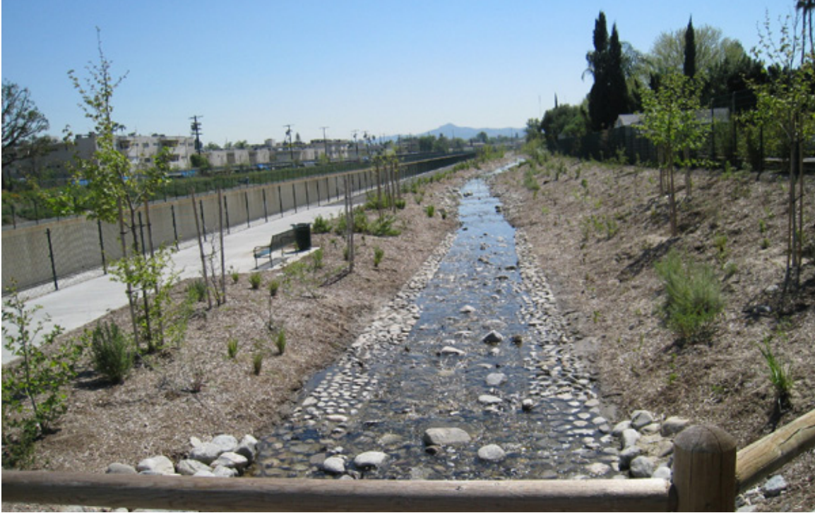
The Tujunga Wash Greenway recreates a historic streambed in Los Angeles. The concrete flood channel (left, beyond the trail) remains in place to handle water from large storms.
