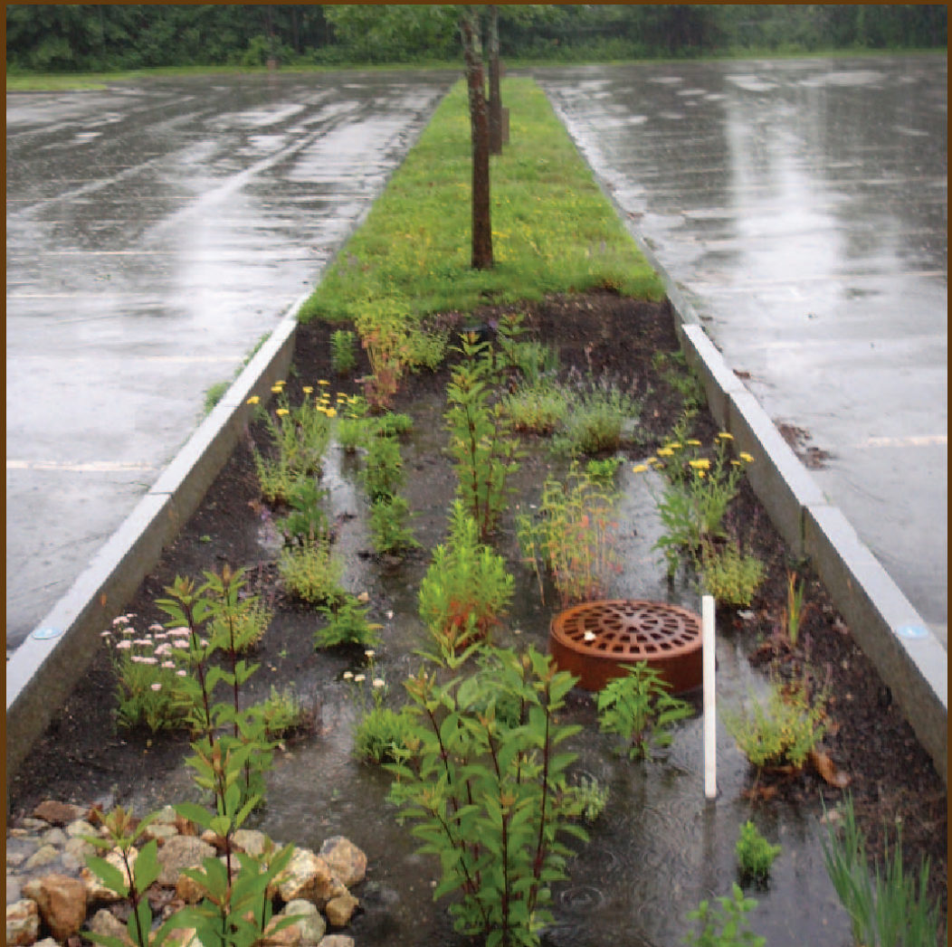
FIGURE 3-5 Completed Bioretention Retrofit Installation 2008
