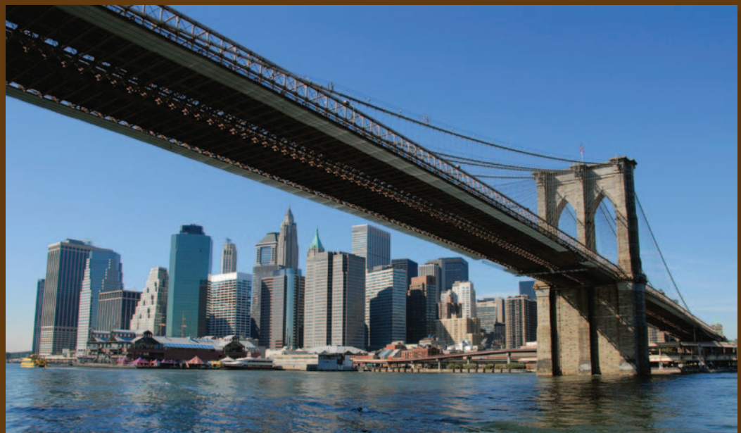
FIGURE 3-12 The Brooklyn Bridge spanning the East River.
