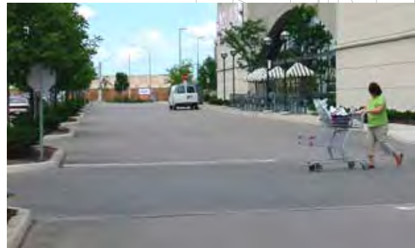
Special pavers define the pedestrian crossing leading to the main building entrance
