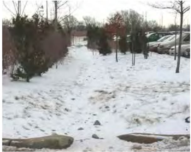
A bio-retention area used for snow storage
