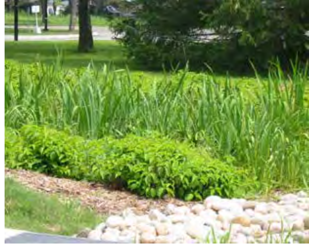
A bio-retention area adjacent to a parking lot drive aisle
