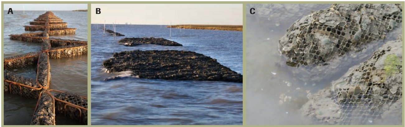
Figure 15. (a) Oyster reefs constructed of metal shell containment units in Mobile Bay, AL. (b) Bagged oyster shell near Dauphin Island, AL. (c) A close up of reef constructed of bagged oyster shell.
