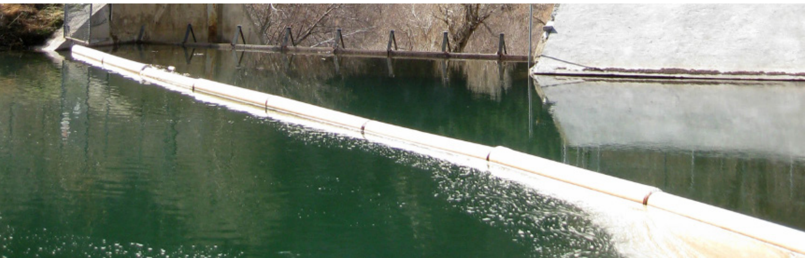
Stairs Gulch penstock intake, Big Cottonwood Canyon. Photo: Tim Bardsley.
