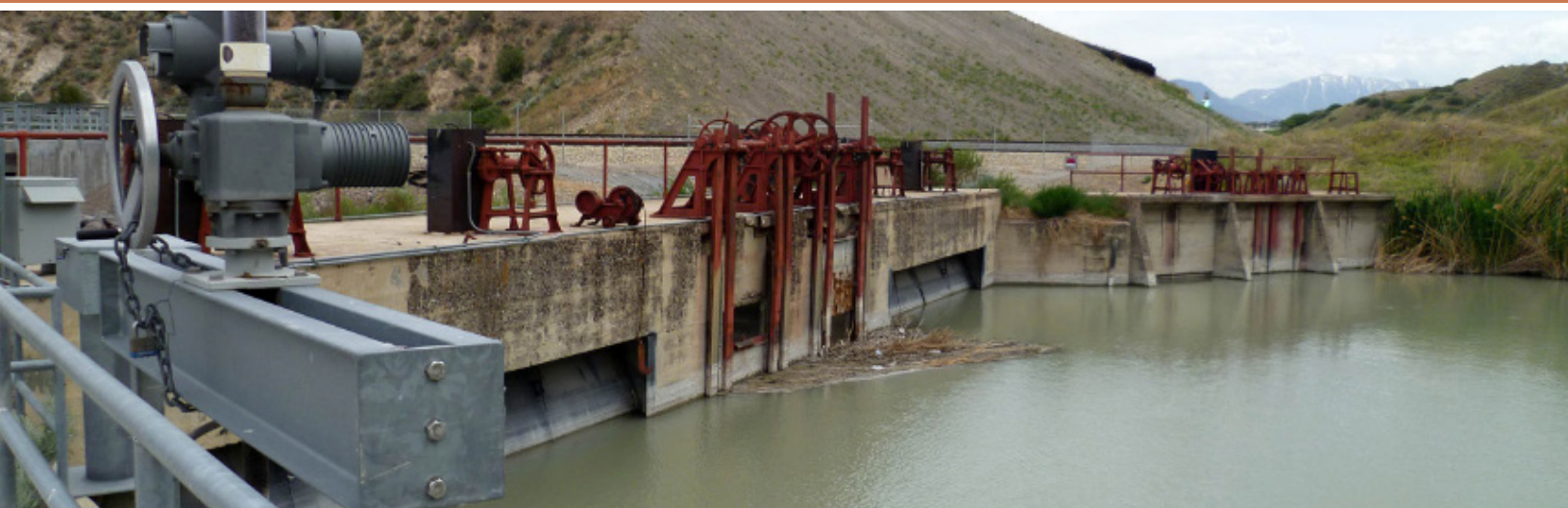
Turner Dam, Jordan River (diverts water to the Utah and Salt Lake Canal on the west side, and the East Jordan Canal on the east side.) Photo: Tim Bardsley.
