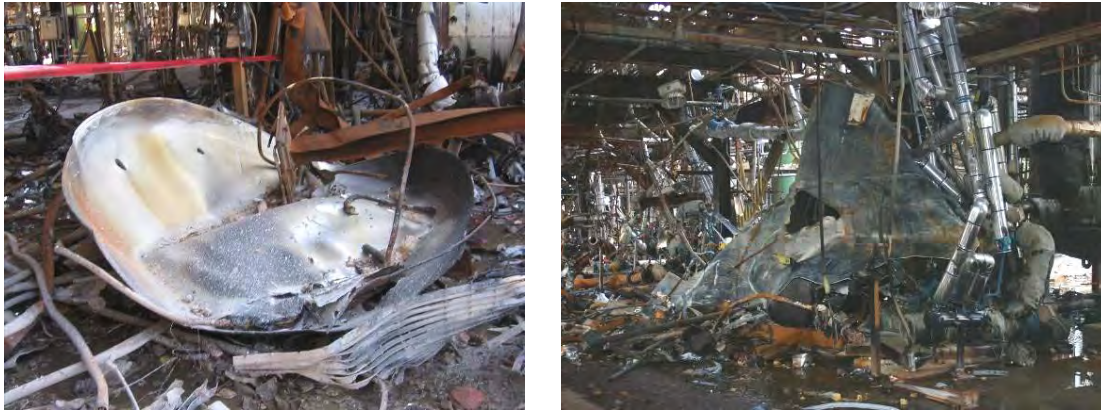
Figure 12. Residue treater bottom head (left); vessel shell and top head (right)
