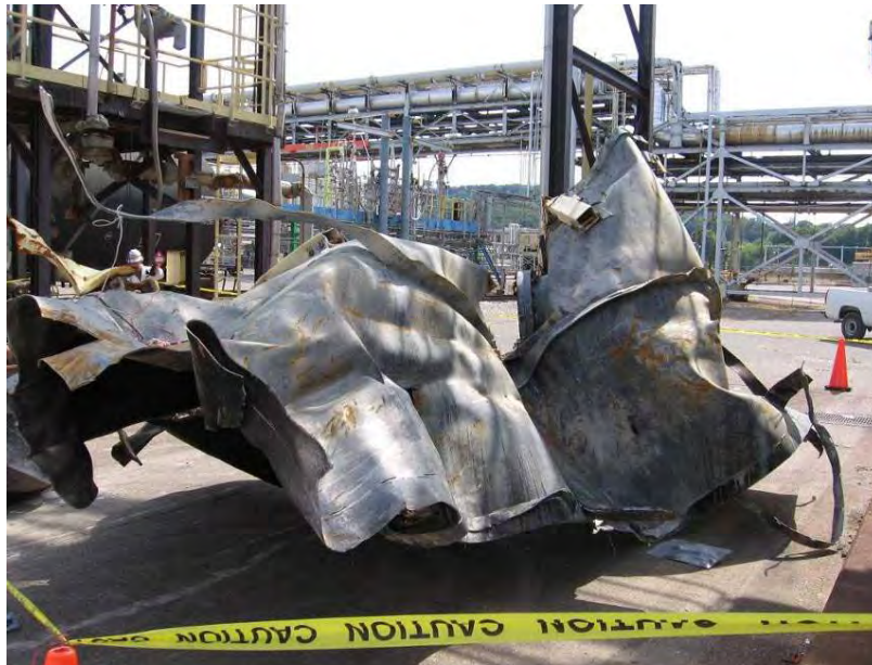
Figure 13. Residue treater shell and top head recovered from inside the Methomyl-Larvin unit
