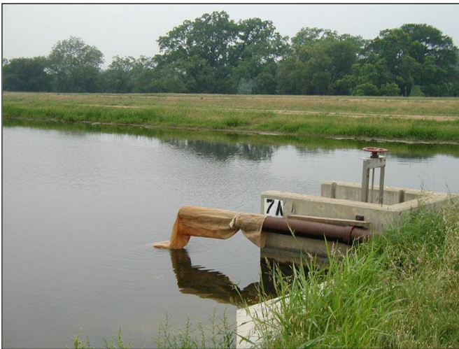
Filtering "sock" on pond water supply line. Photo Credit: Bob Pitman & Robert Lindsey, USFWS
