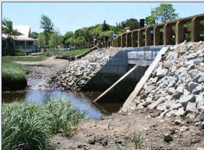
Figure 16. NRCS provided funding to replace an undersized culvert with a new box culvert, restoring 65 acres of Sesuit Creek salt marsh in Dennis, Massachusetts. Source: NRCS, 2008b.
