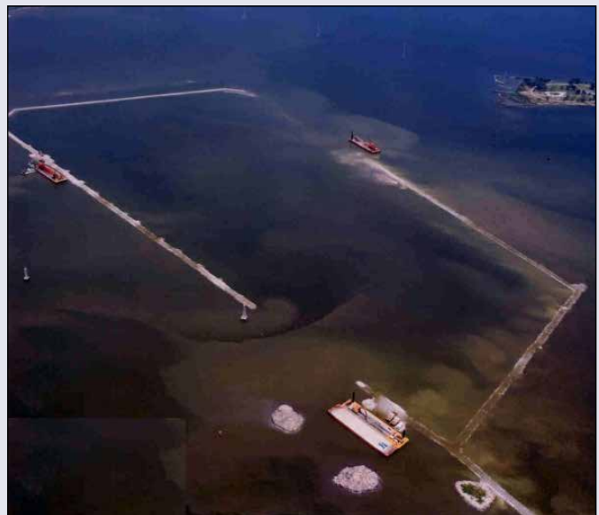
Figure 12. Dredged material was used to restore Goat Island, seen here in an intermediate stage of restoration. Photo courtesy of Beneficial Use Group.
