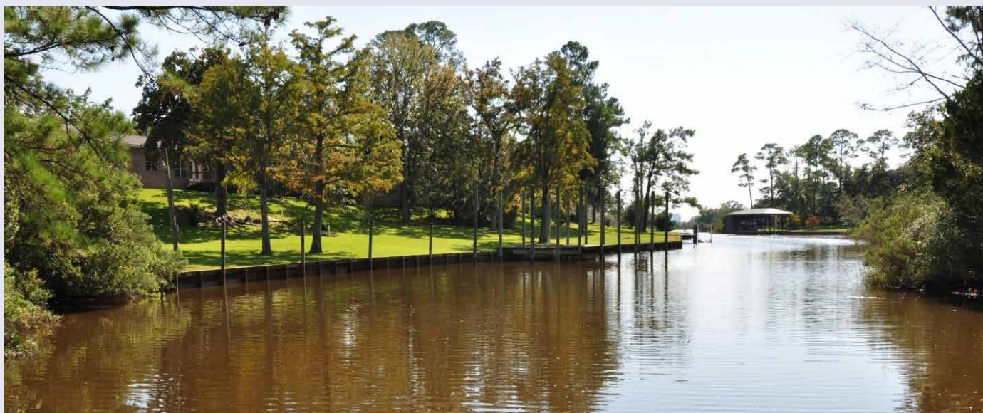
Figure 22. Gulf Hills, an example of a subdivision with extensive bulkheading. Photo courtesy of Martina McPherson, ERG.
