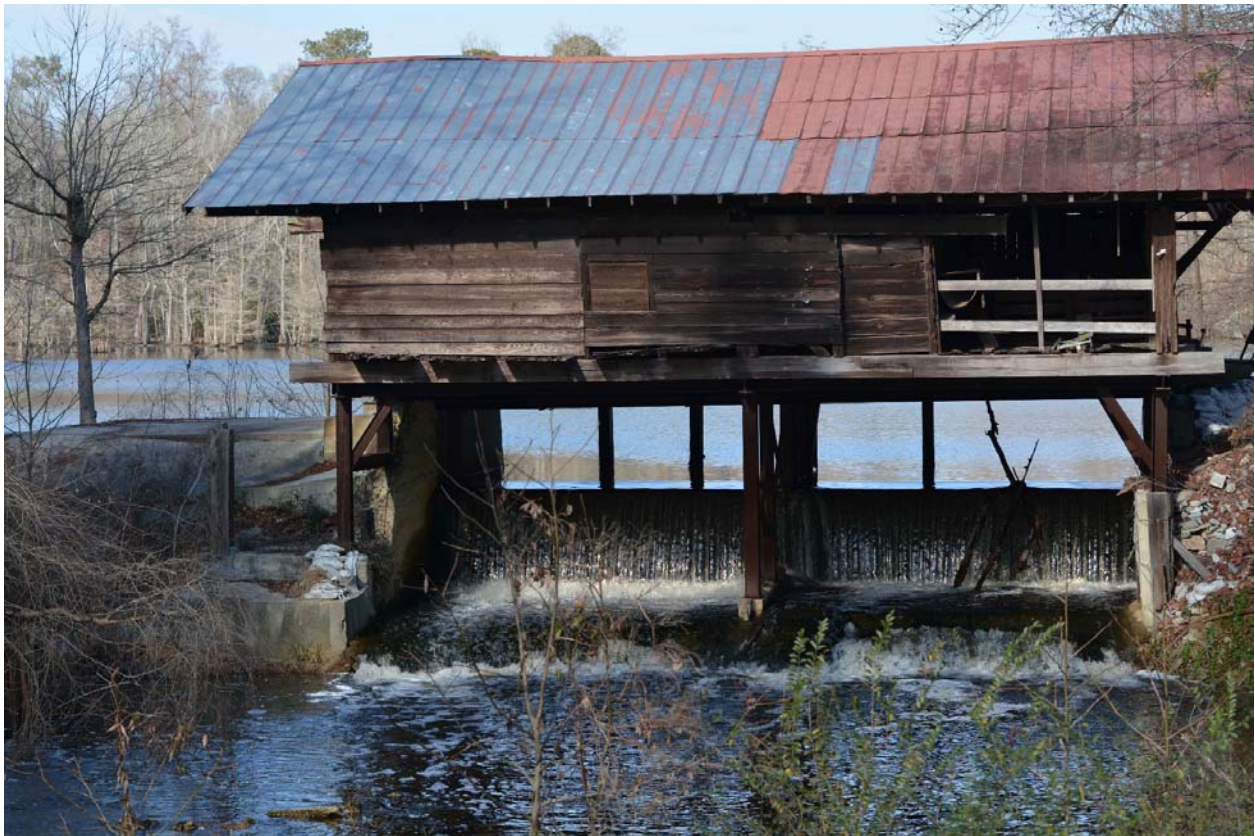
Boney Millpond Dam, natural barrier may make this a low priority. Photo by Fritz Rohde
